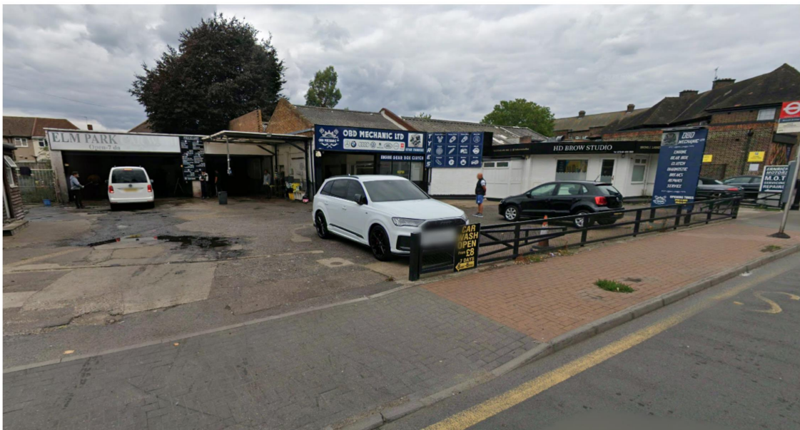
Figure 3: garages at 235-243 Elm Park Road (source: Google Maps)
