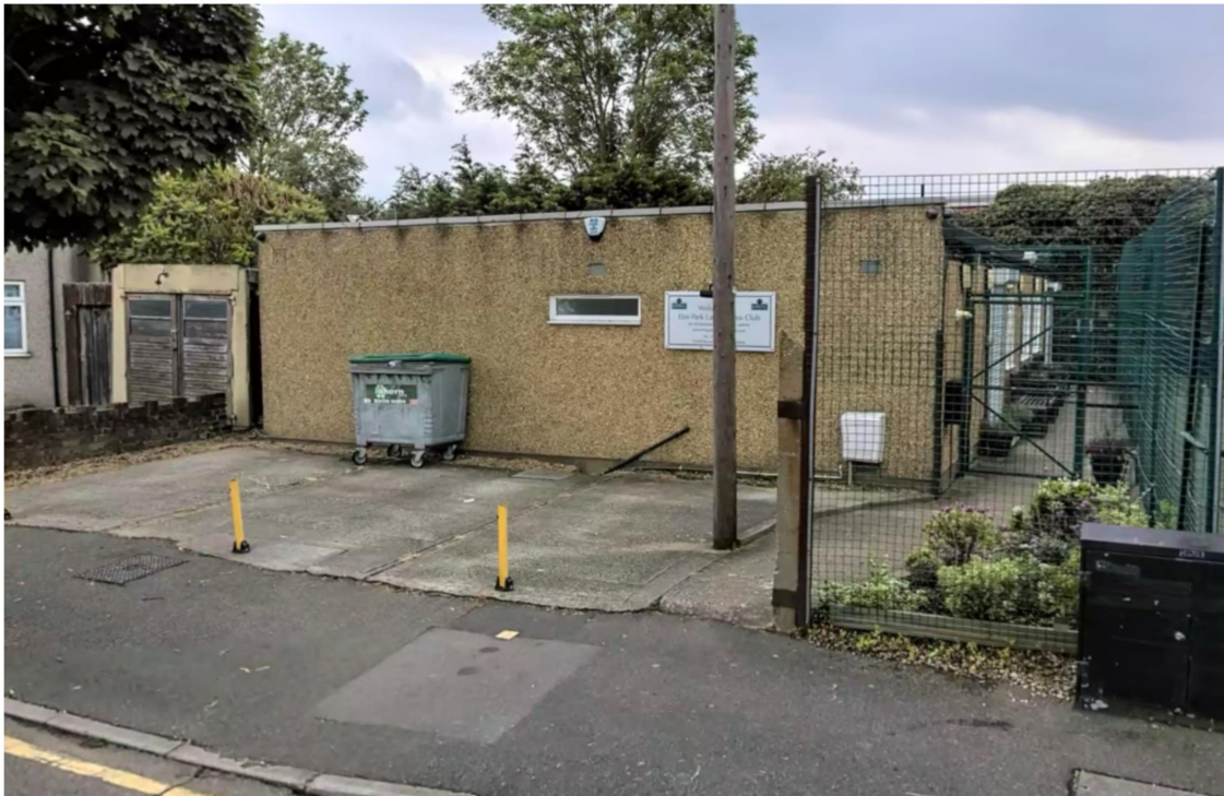
Figure 2: Elm Park Lawn Tennis Club building (source: Apple Maps)
