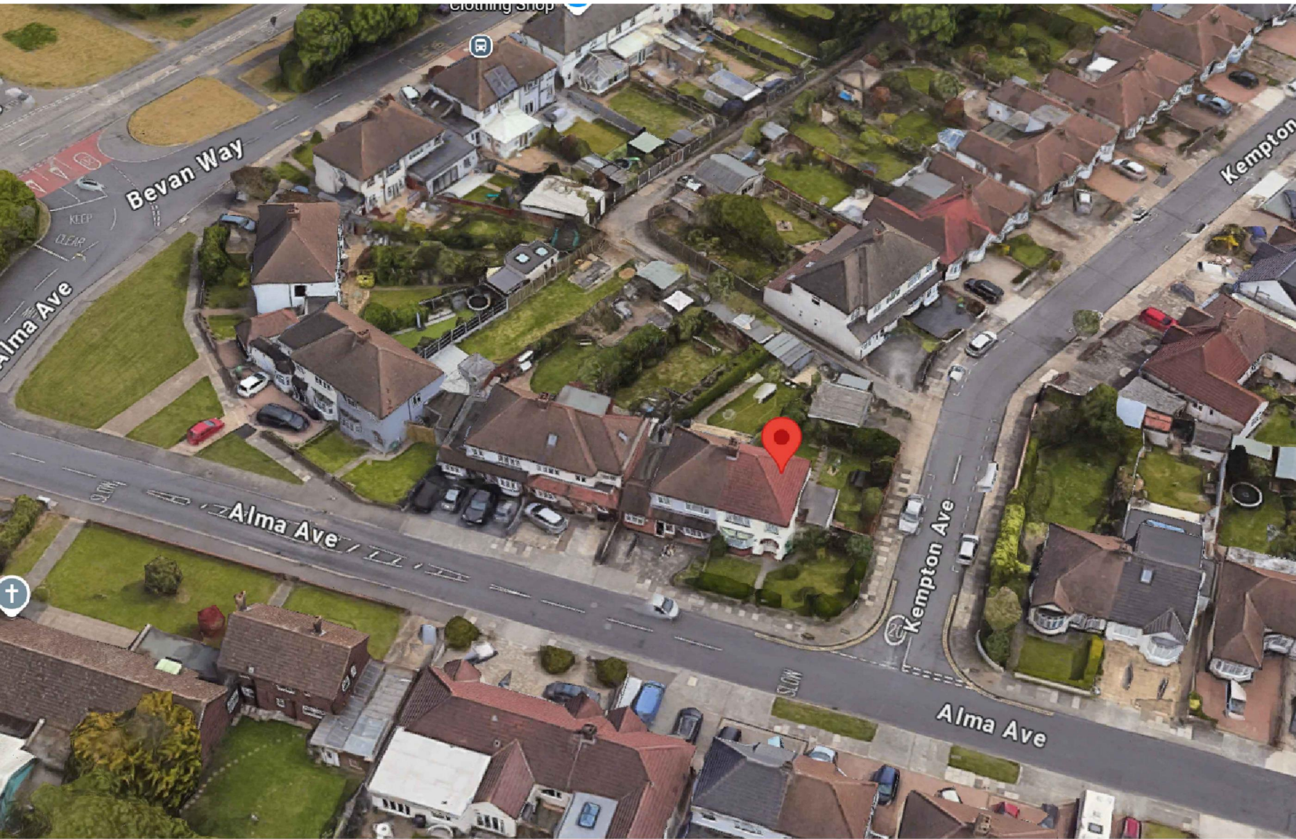
04 AERIAL PHOTOGRAPH N.T.S.
