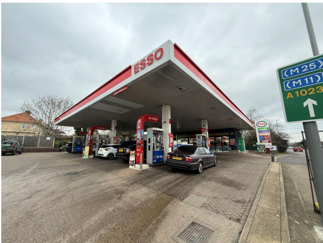
Photo 6: Hardstanding covers the forecourt and building B1 which is assessed as negligible potential for bats.
