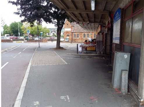
Photograph 3: u1b built structures
