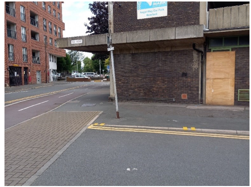
Photograph 2: u1b built structures
