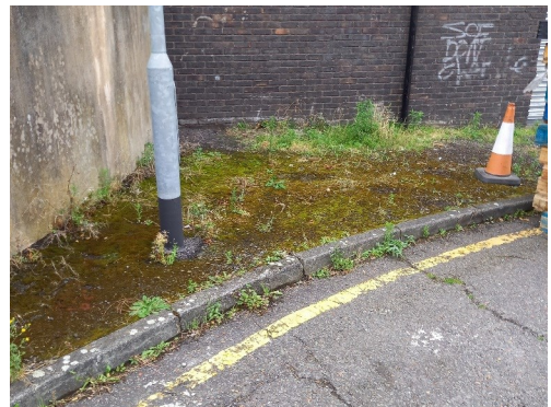
Photograph 6: u1b built structures
