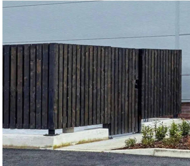
Reference photo for Bin Store Enclosure
