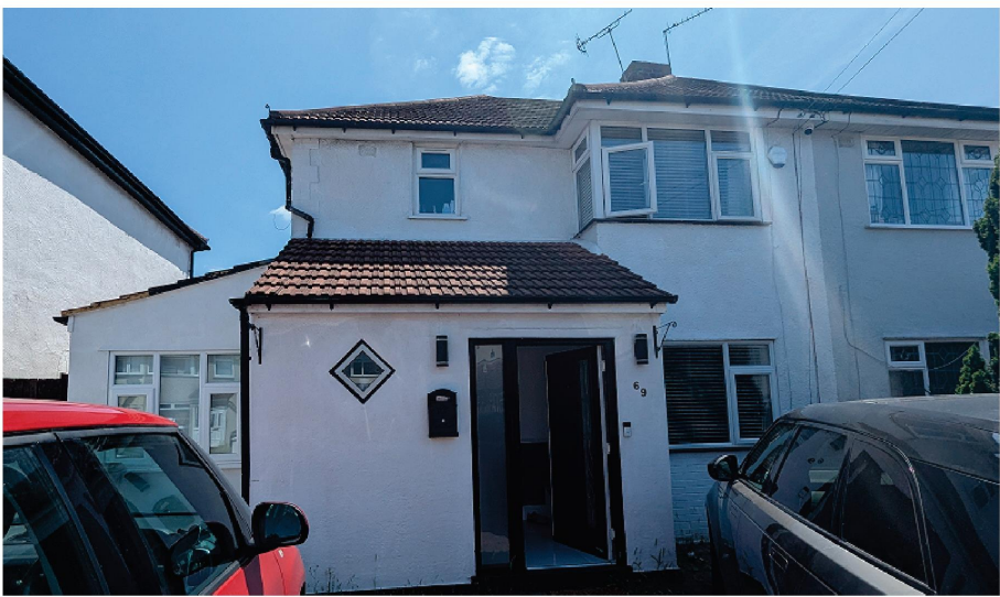
PHOTO - EXISTING FRONT ELEVATION
