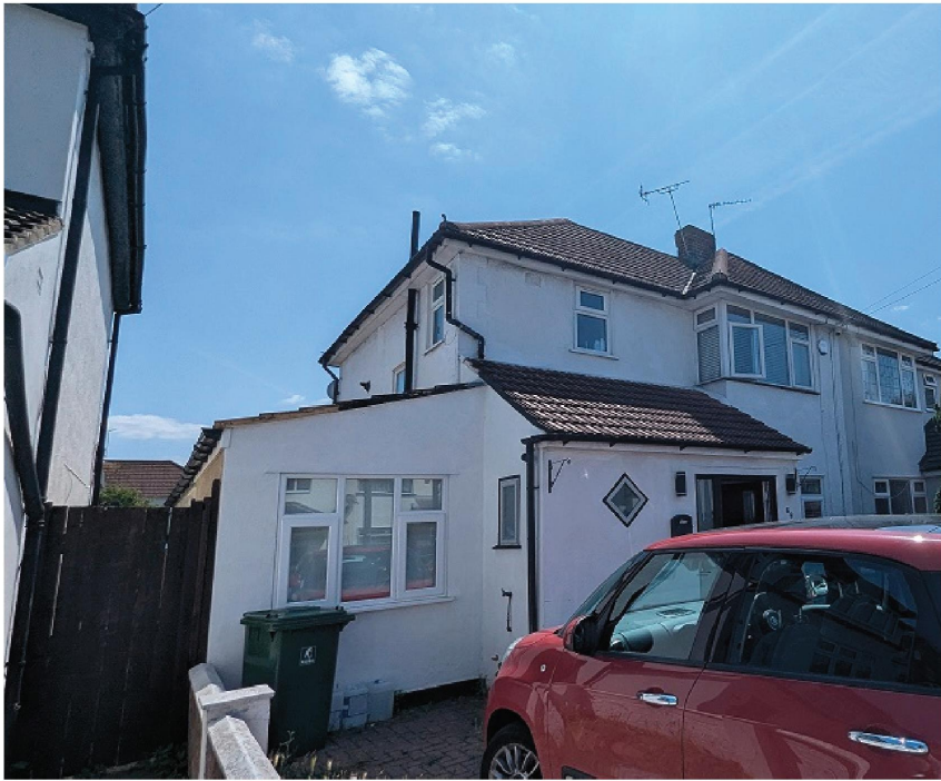
PHOTO - EXISTING SIDE ELEVATION
