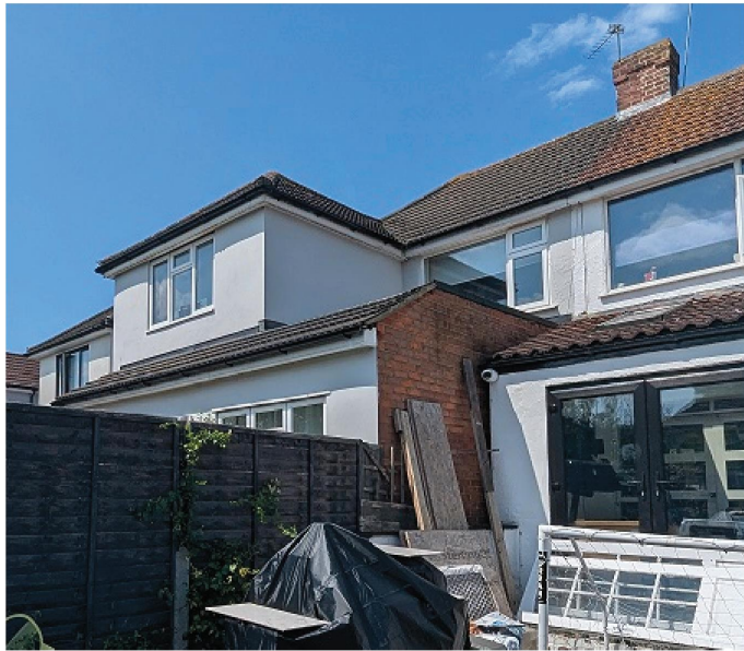
VIEW AT THE NEIGHBOURING PROPERTY 71 CALBOURNE AVENUE
