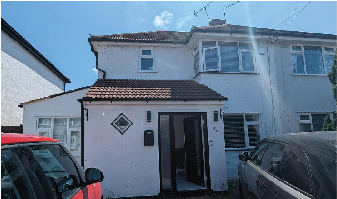
PHOTO - EXISTING FRONT ELEVATION
