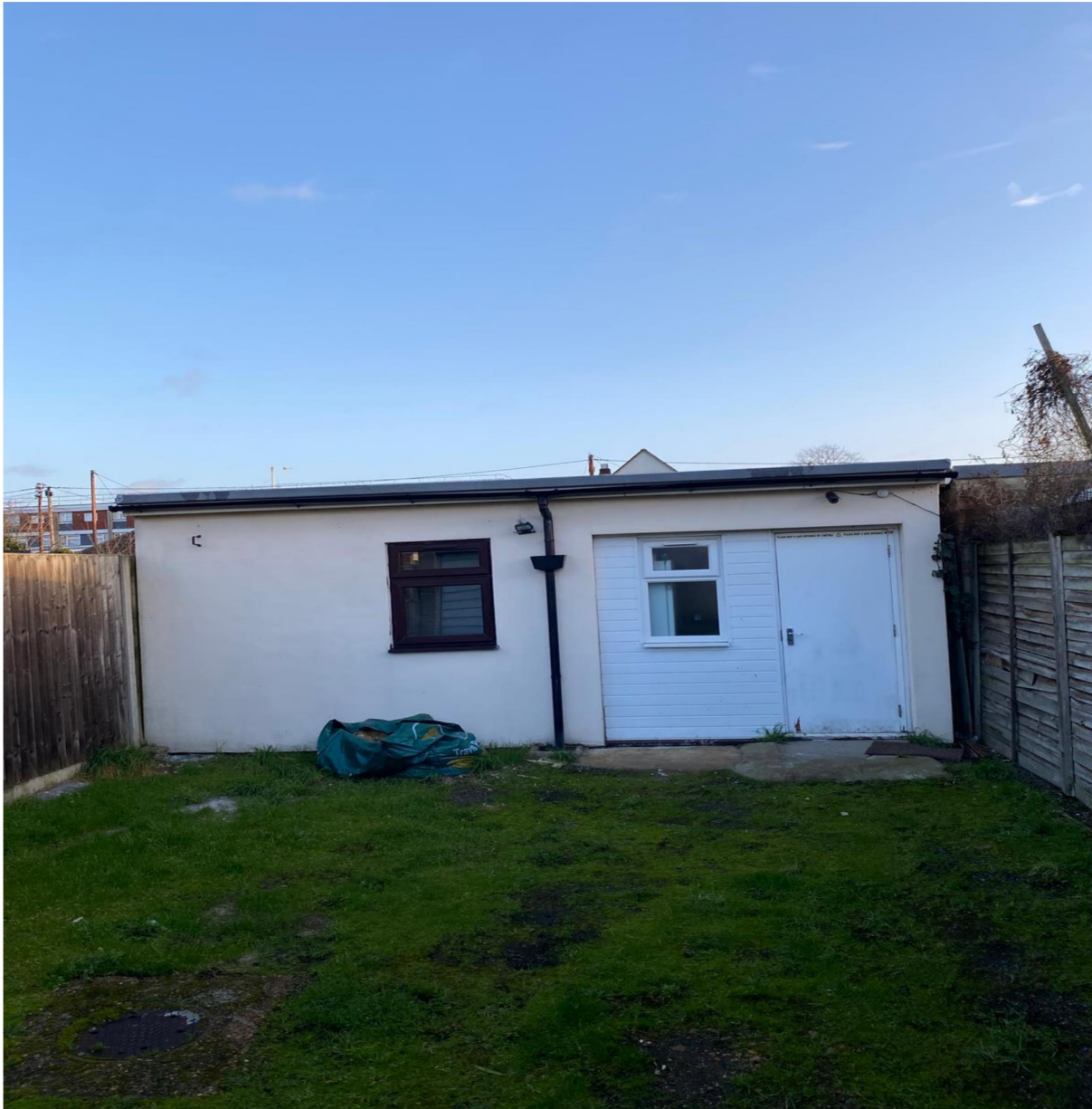
Image 3: View of rear elevation with outbuilding.
