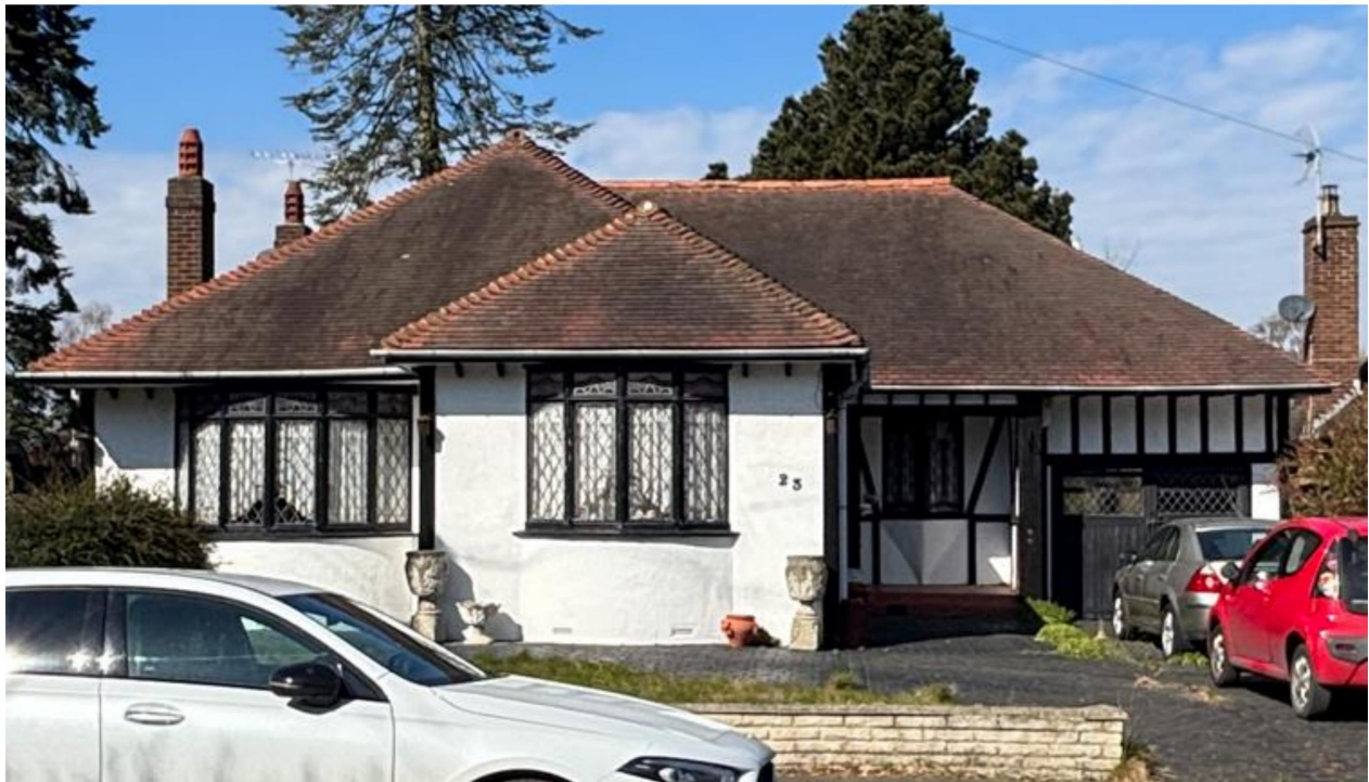
Photo (Courtesy A & P Designs Ltd.) front elevation.
