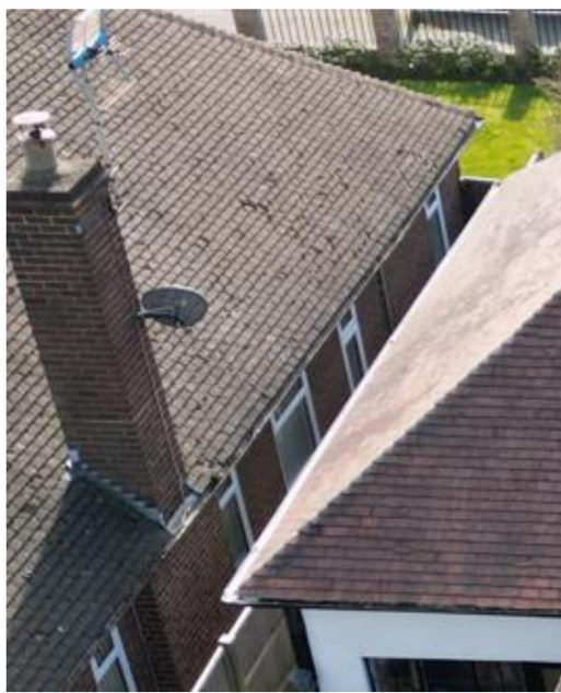
Existing boundary between no 23 and 25 very little sunlight penetrates between the properties as existing.
