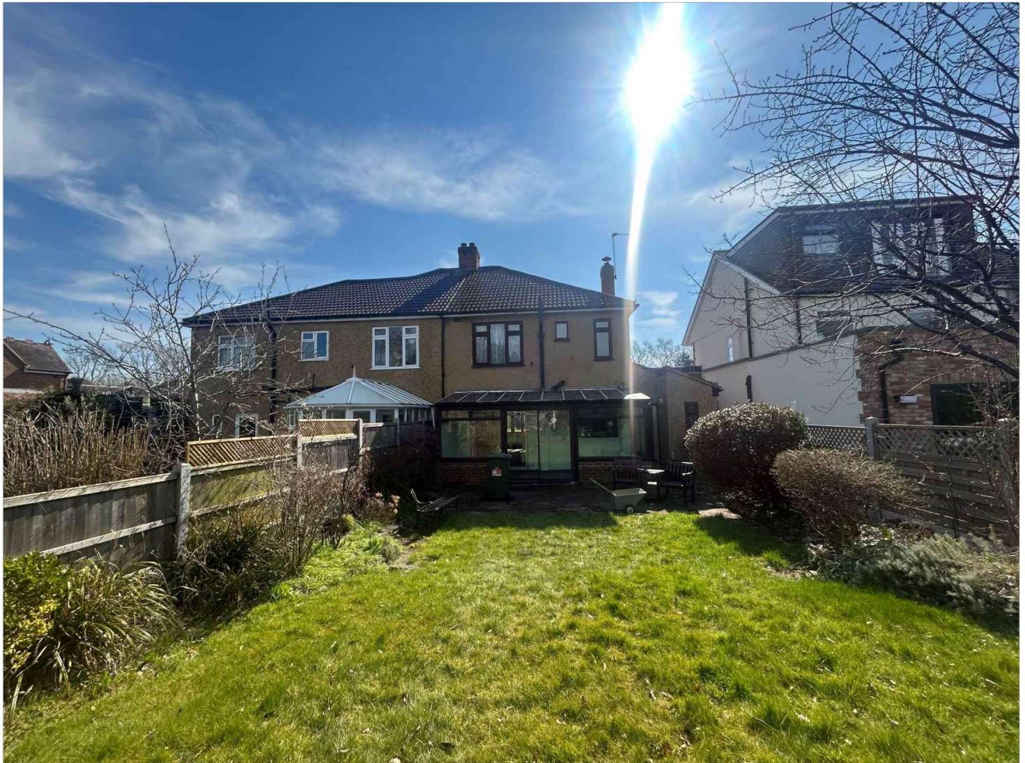
07 REAR PHOTOGRAPH N.T.S.
