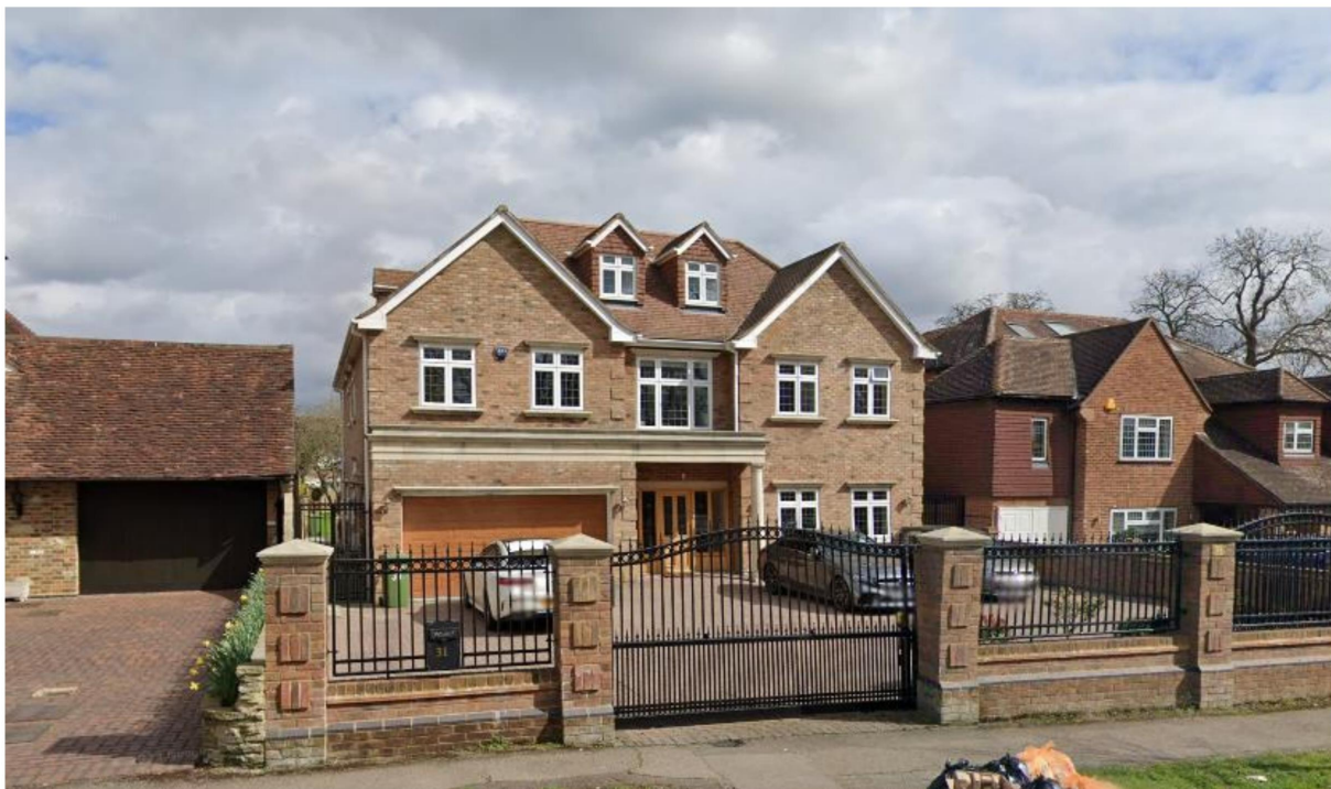
Picture 3. Nelmes Way: Newly built dwelling with double front gable with two front dormers (with integral garage)
