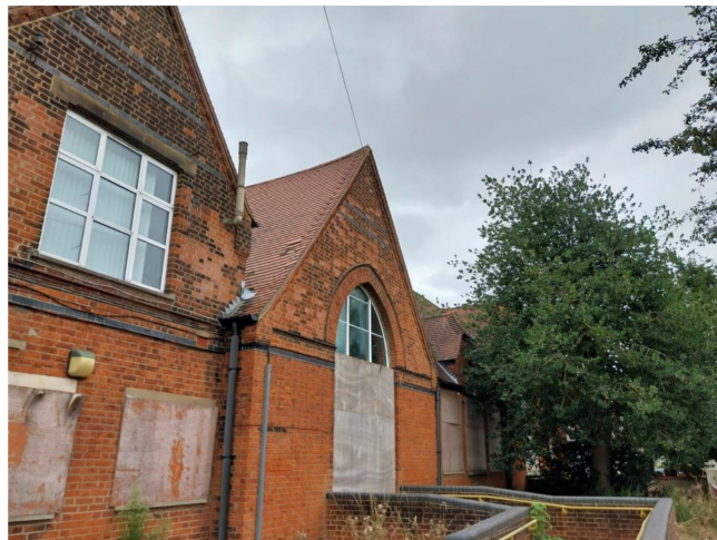
Photograph 2: West (street side) of the main school building (B1). T1 can be seen to the right.
