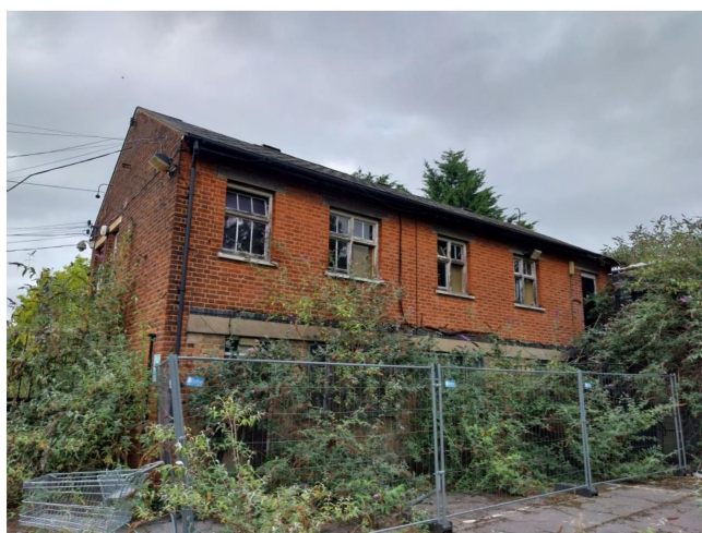
Photograph 3: Building 3 (B3) surrounded by scattered buddleia scrub.
