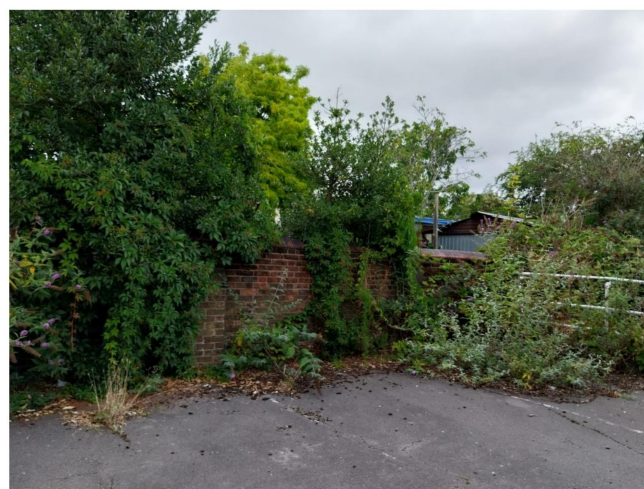
Photograph 10: INNS Virginia creeper (TN2) located on site climbing over the boundary wall.
