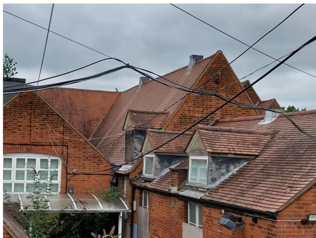
Photograph 5: Back of Building 1 (B1) with an example of the com- plex roof structure.
