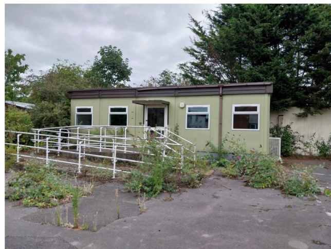
Photograph 6: Building 4 (B4) showing a prefabricated cabin build- ing.
