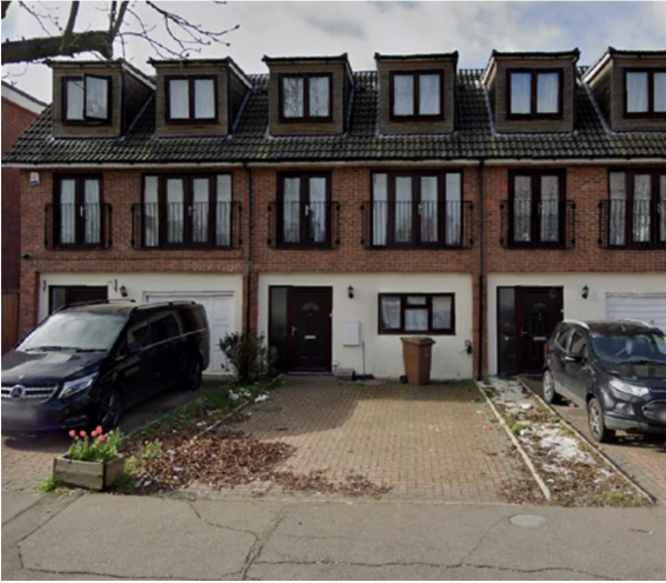
Existing Parking Area
