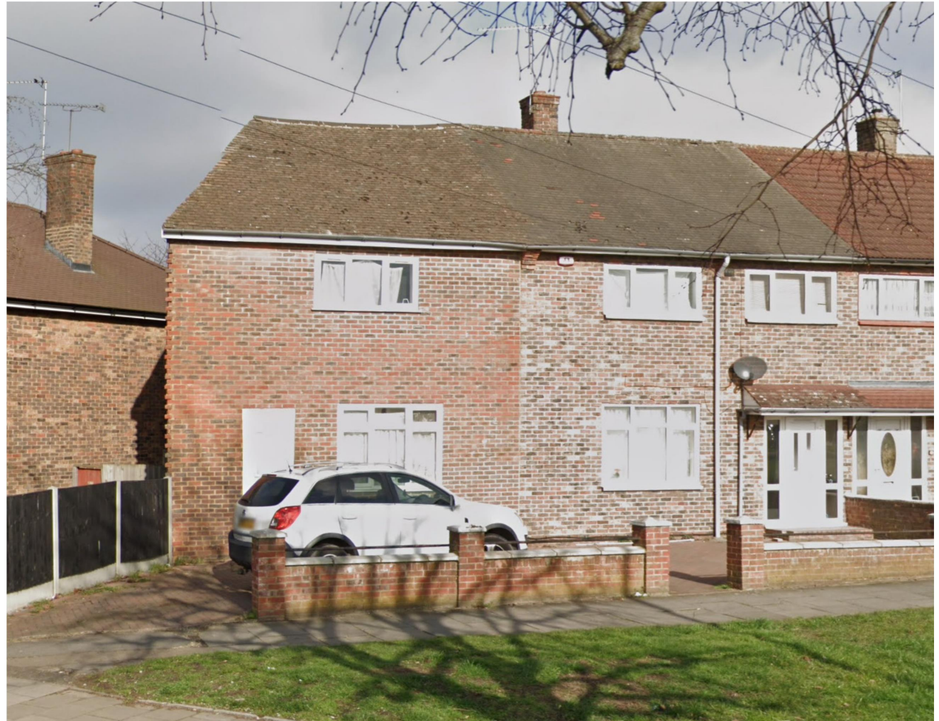
Photograph of Existing Front Elevation
