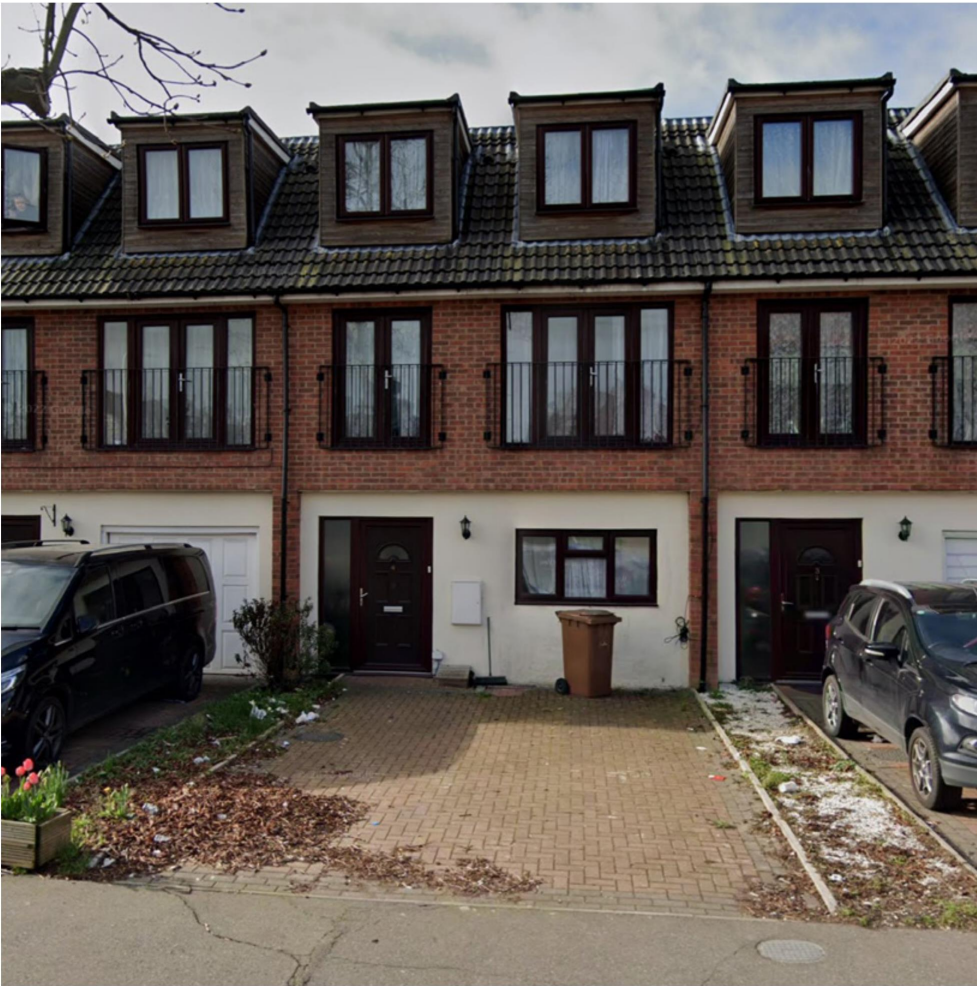
Front Elevation (showing the primary access to the property)
