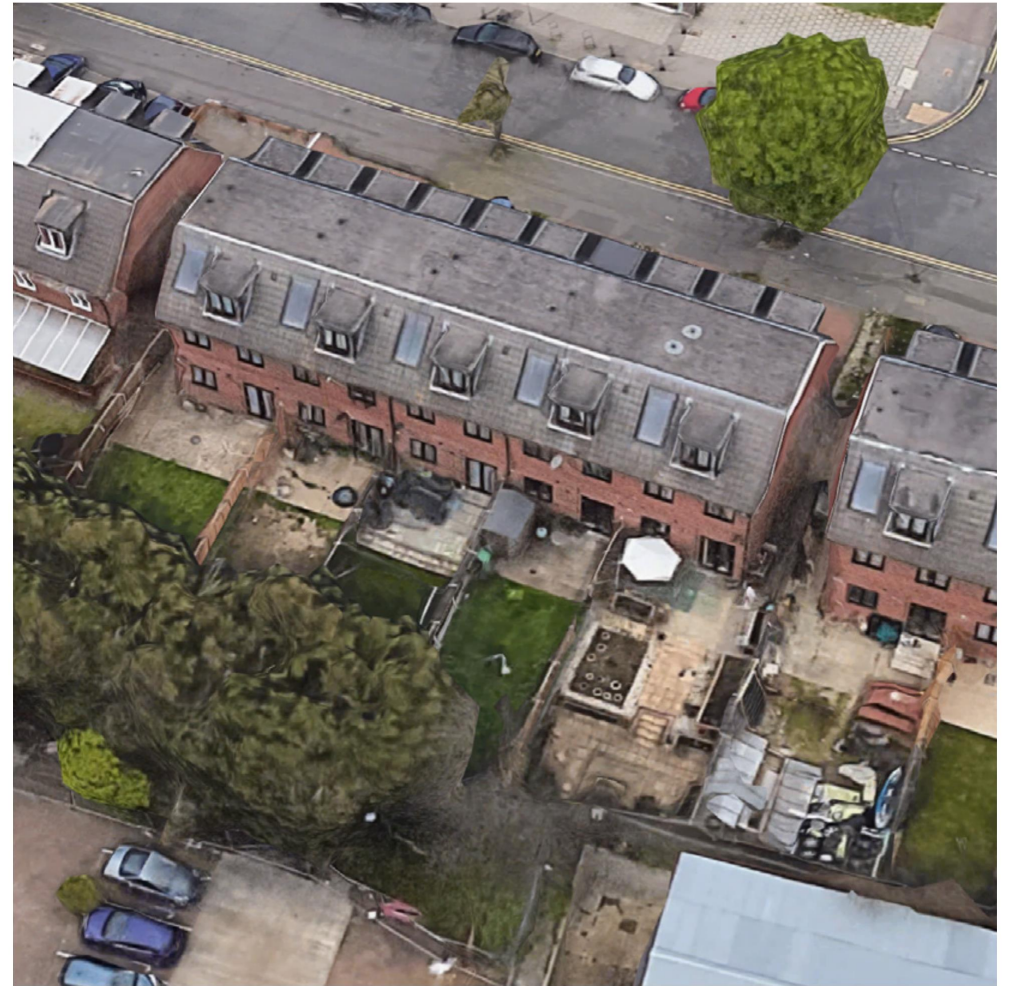
Aerial Photograph Showing Rear Elevation
