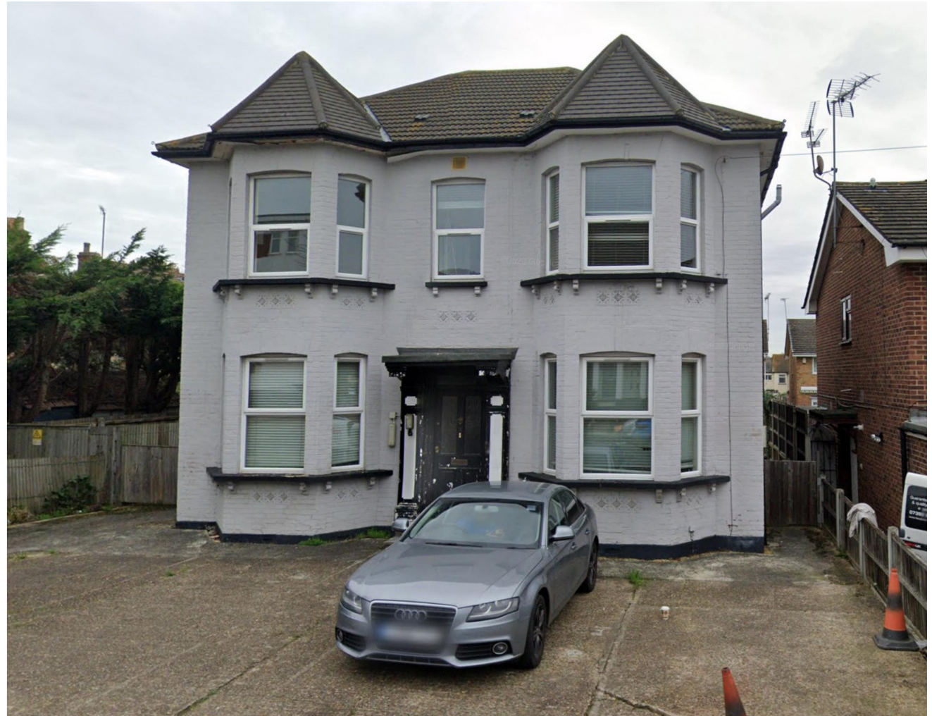
Photograph of Existing Front Elevation
