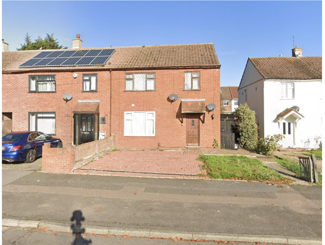
Photograph of Existing Front Elevation
