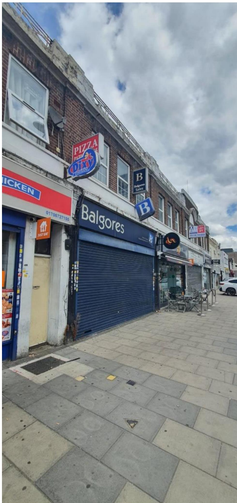
Front view to site (Balgores)
