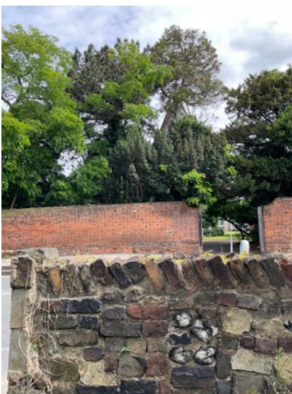
Photograph of the low church wall and C18th chaplaincy wall behind (looking north from the church)
