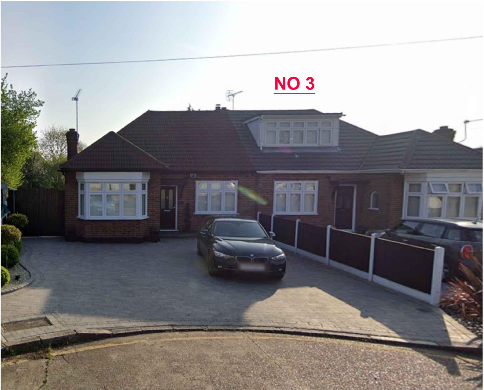
26 PHOTOGRAPH SHOWING EXISTING DORMER AT NO 3 MARIAM GARDENS N.T.S.
