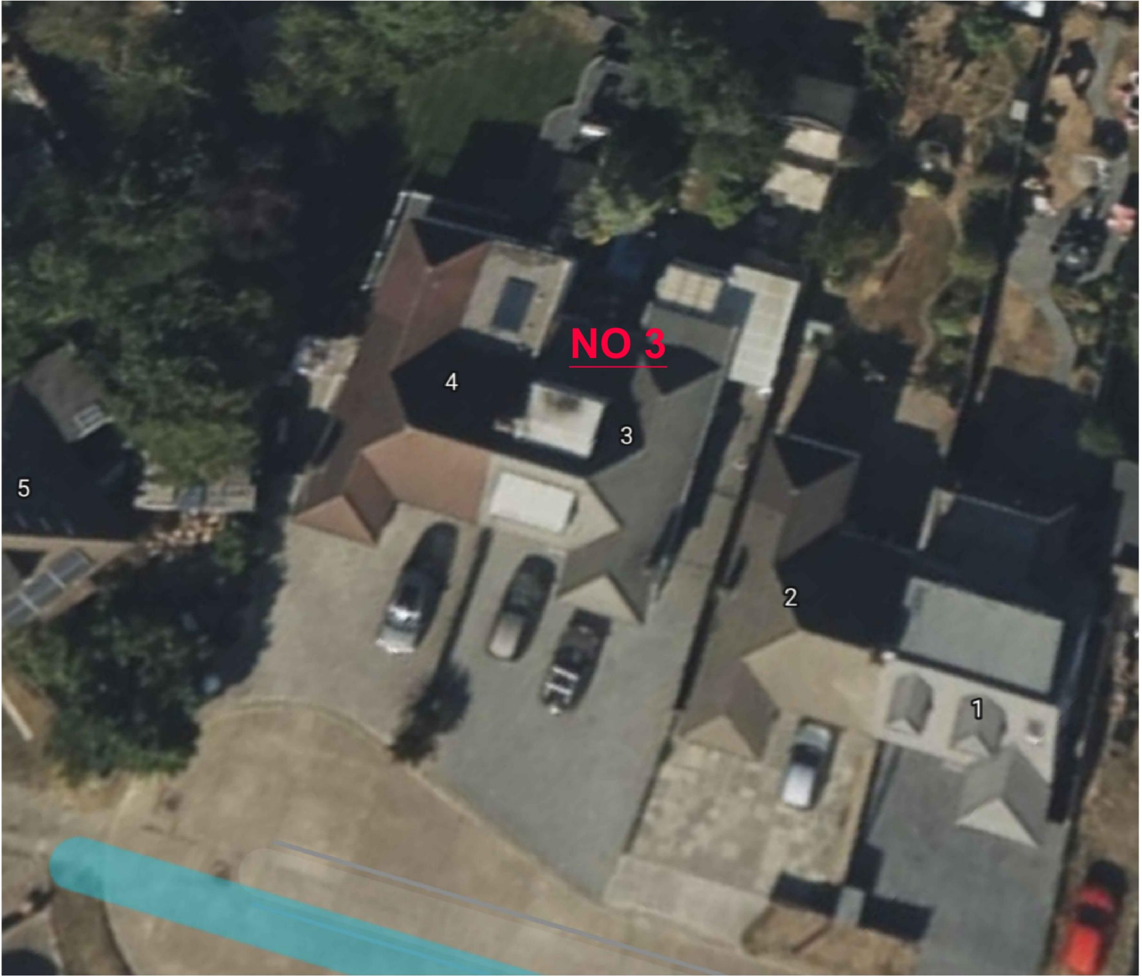
27 AERIAL PHOTOGRAPH SHOWING EXISTING DORMER AT NO 3 MARIAM GARDENS N.T.S.
