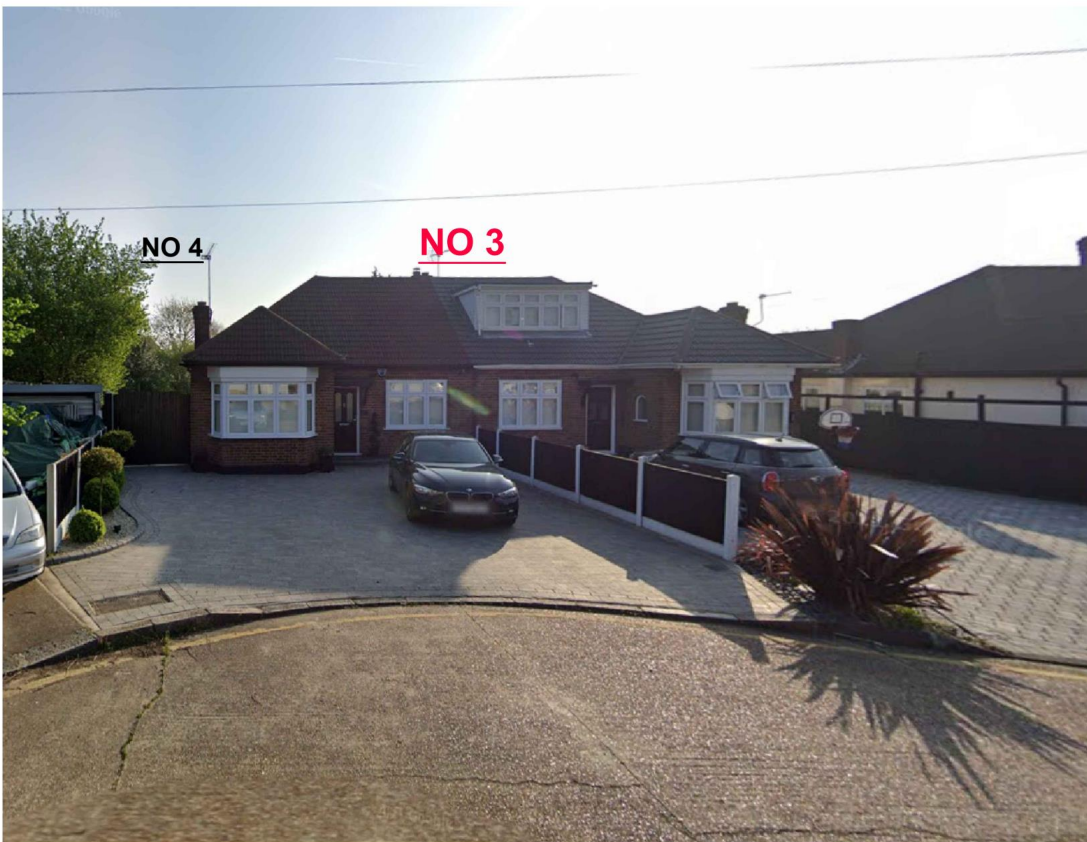
21 PHOTOGRAPH SHOWING EXISTING DORMER AT NO 3 MARIAM GARDENS N.T.S.
