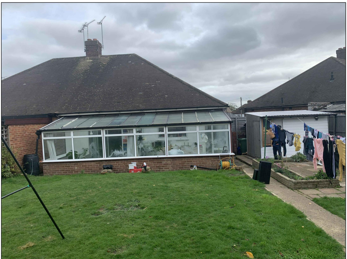
10 REAR PHOTOGRAPH N.T.S.
