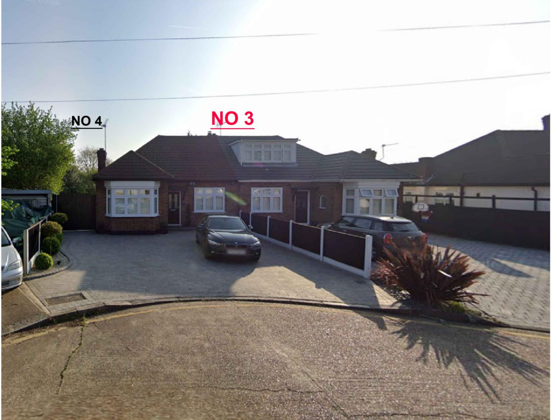
21 PHOTOGRAPH SHOWING EXISTING DORMER AT NO 3 MARIAM GARDENS N.T.S.
