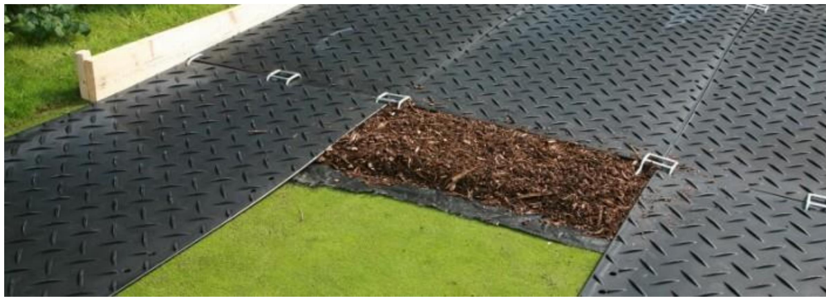
Figure 8. Example of ground protection suitable for pedestrian operated plant up to a gross weight of 2.0t. Interlinked ground protection boards which are laid on top of a layer of woodchip with geotextile membrane below.
