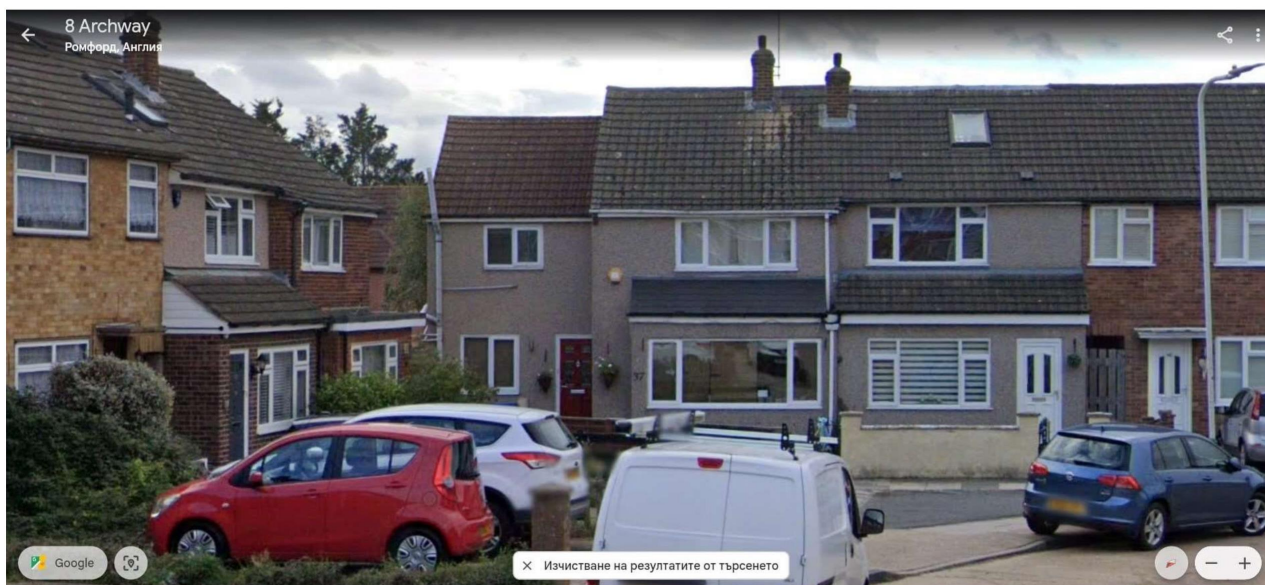
Street Elevation looking north onto Archway (37 Archway end of terrace on the left)
