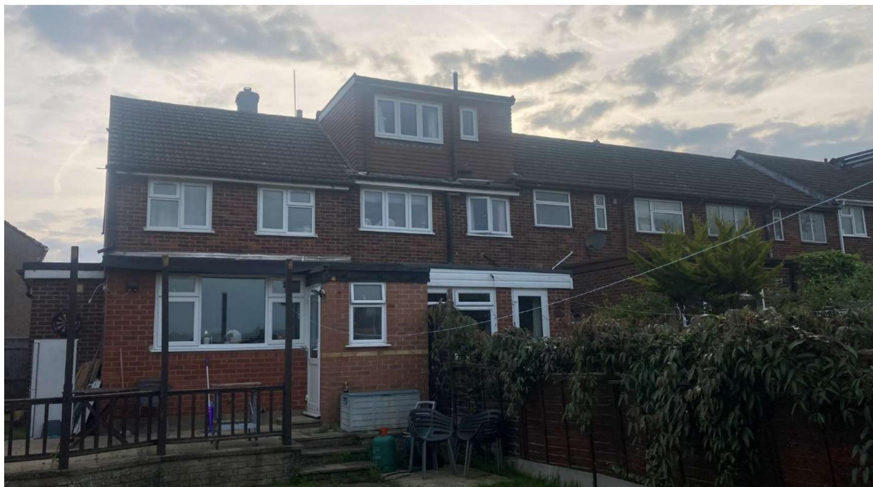
Existing Rear Elevation of 35 Archway with 33 Archway to the right
