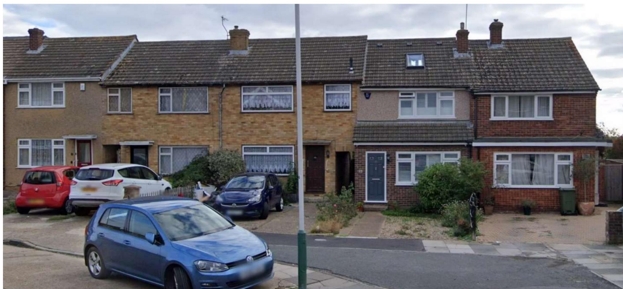
Street Elevation looking west onto Archway (35 Archway end of terrace on the right)
