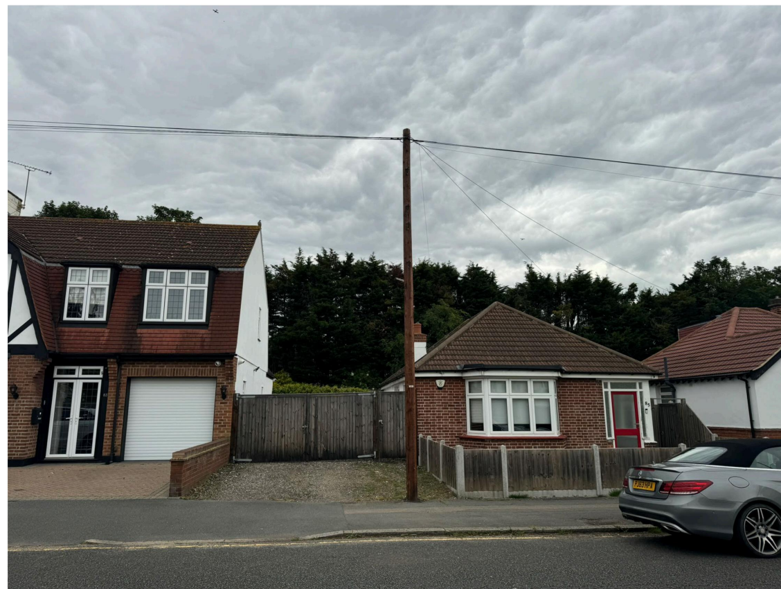
P2. Photo showing front elevation of 85 Howard Road.
