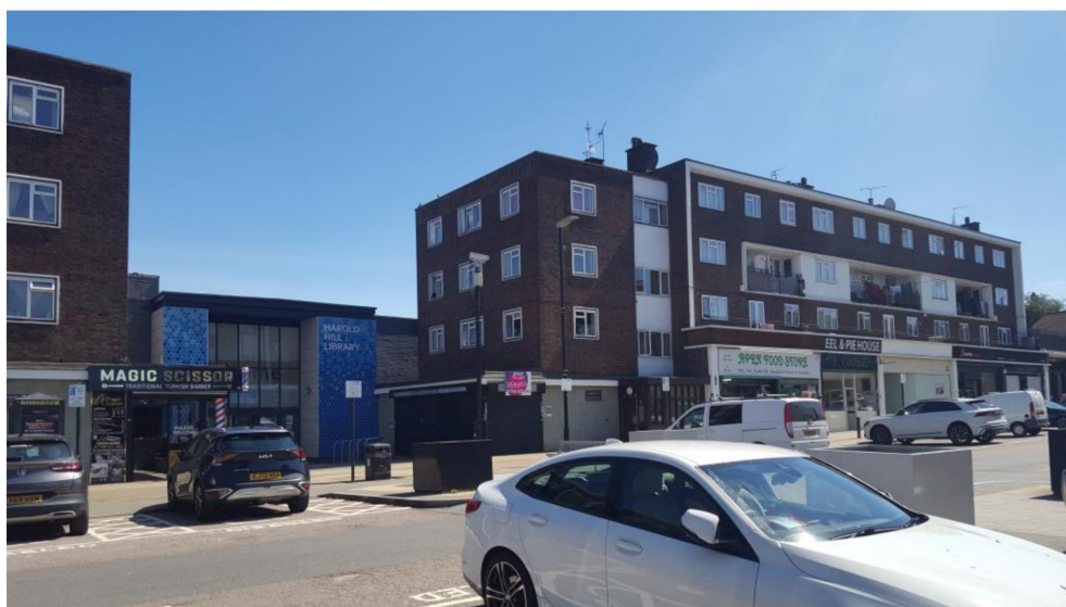
Photograph 2 - Rear of 4-storey blocks with commercial buildings at ground level
