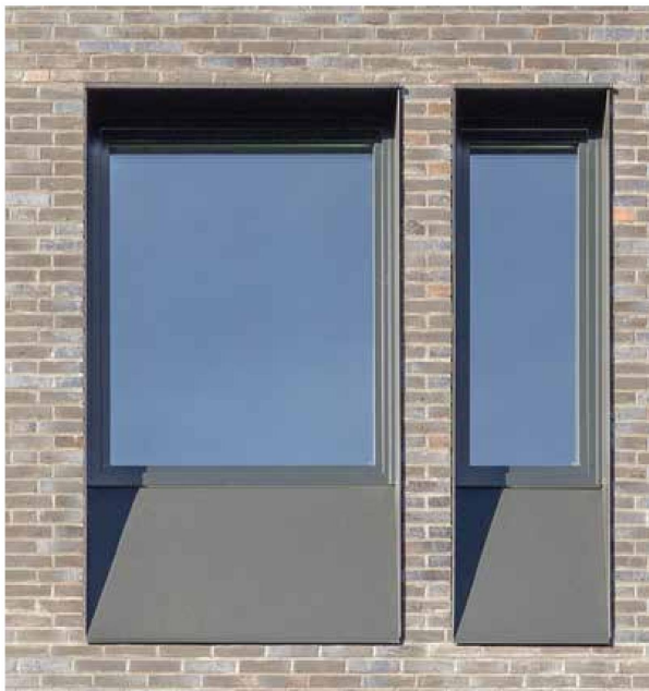
G-02 WINDOWS RECESSED IN METAL PANEL FRAME
