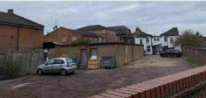
2 Rear of Site seen from the north
