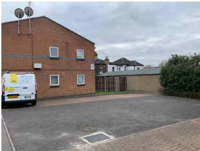
6 Boundary wall from Corbridge Mews
