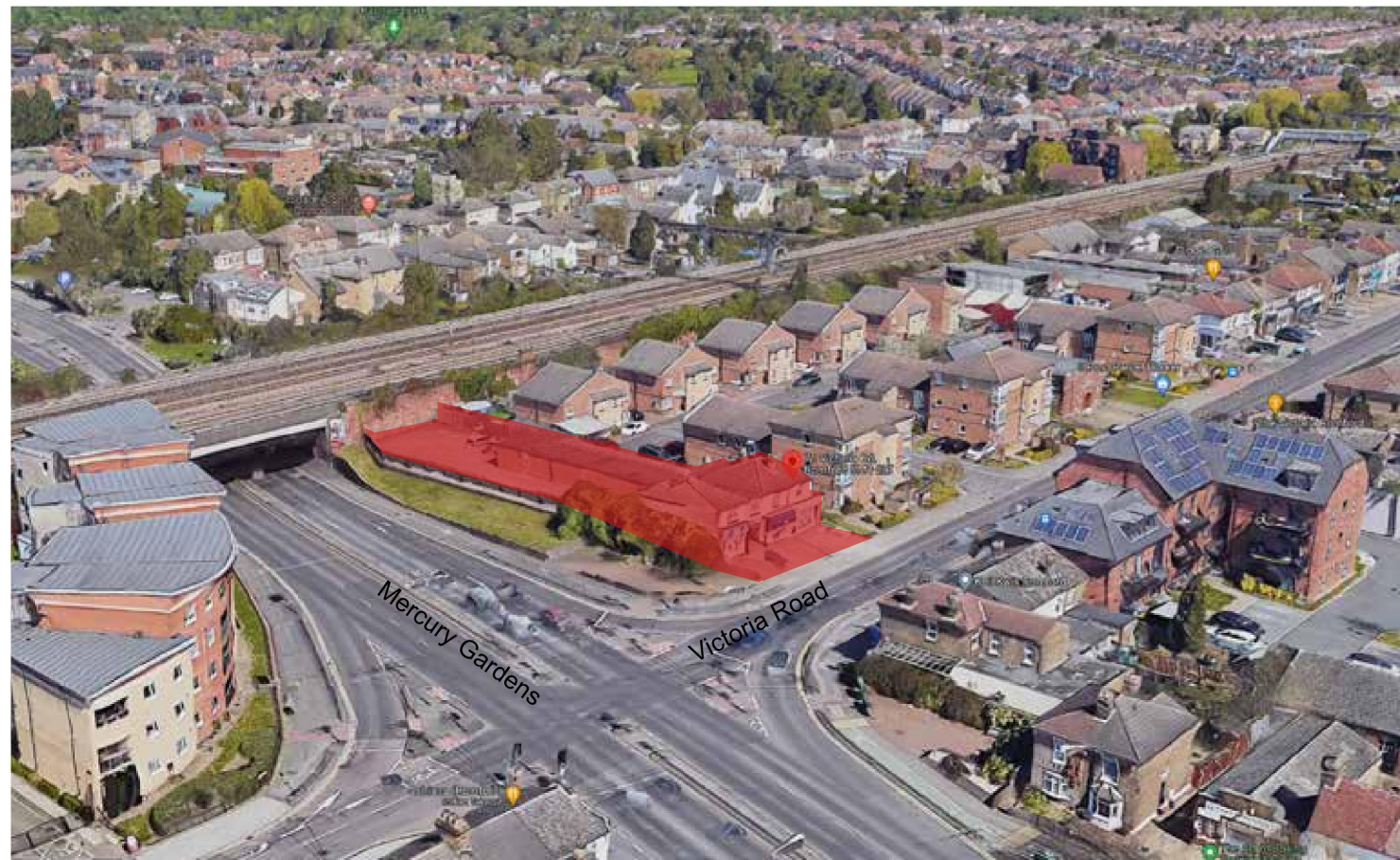
Aerial View From Southwest
