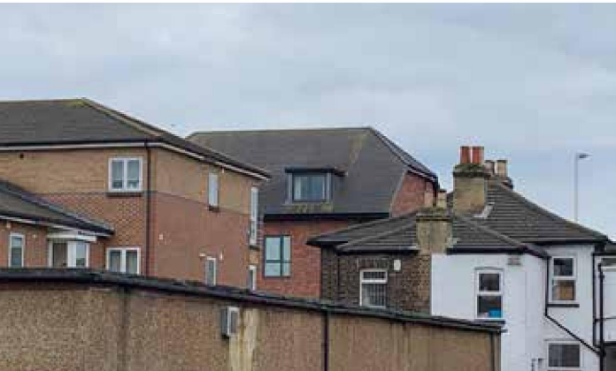
3 Rear of Buildings
