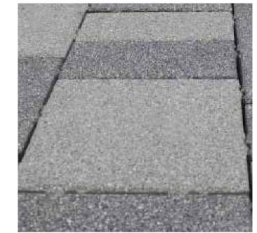
Permeable concrete flag paving
