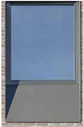
G-02 WINDOWS RECESSED IN METAL PANEL FRAME
