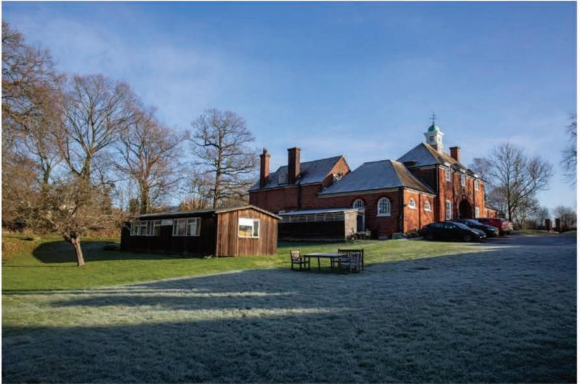
Plate 7. Upminster Court stables and adjacent pre-fabricated building, looking northeast
