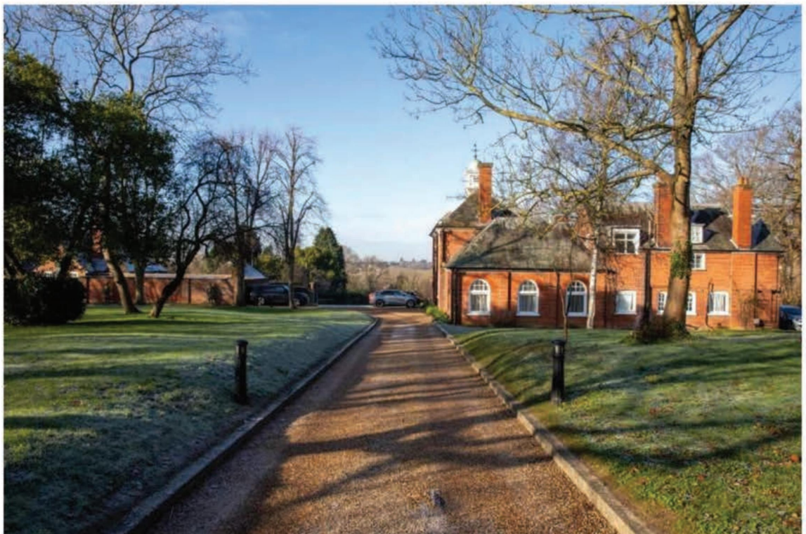
Plate 4. Upminster Court stables driveway access, looking west within gardens
