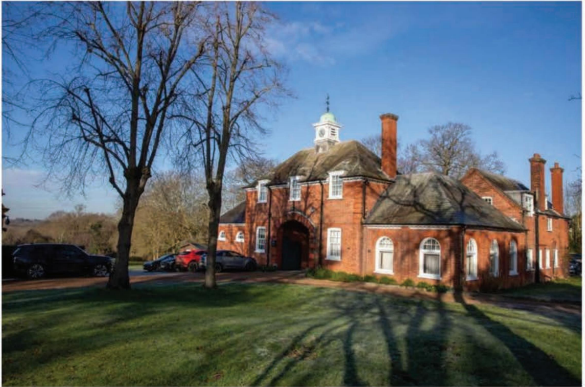
Plate 5. Upminster Court stables front and side elevations, looking northwest from front lawn
