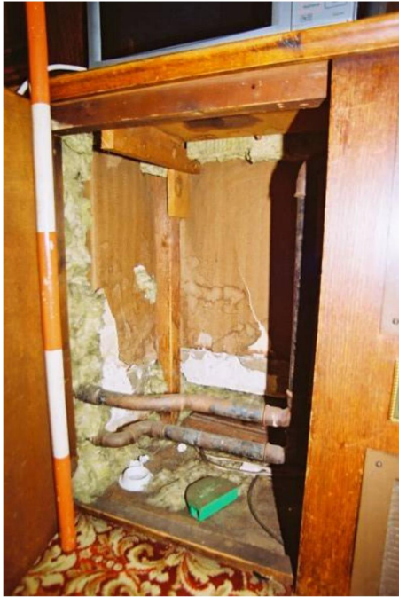
Figure 15 Pre-panelling wallpaper of the east wing (F1:12)
