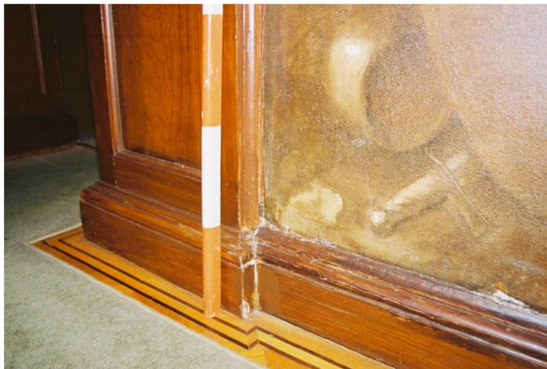
Figure 12 Renewed and original skirting board below the wall painting at first-floor level (F1:18)
