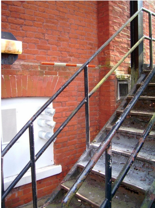
Figure 6 Building break between Maintenance Office and Laundry Room (F2:30)
