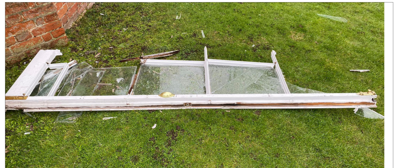
Figure 4. ExD06, detached door leaf after storm in January 2024.
