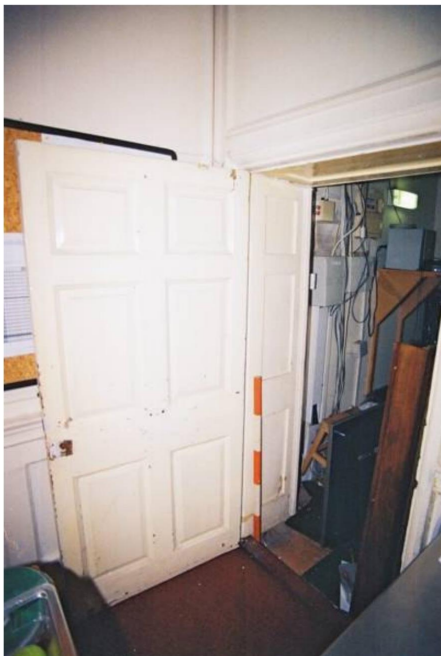
Figure 9 The north-east 'Serving'; 1730 entrance to passage
