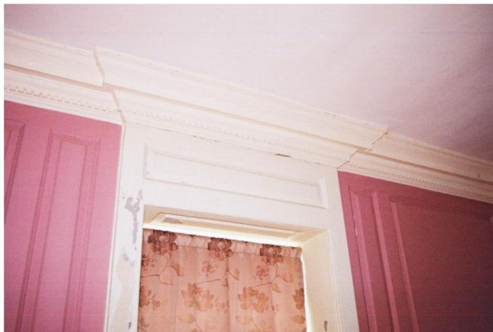
Figure 18 The south-west bedchamber; elaborate panelling (F1:20)
