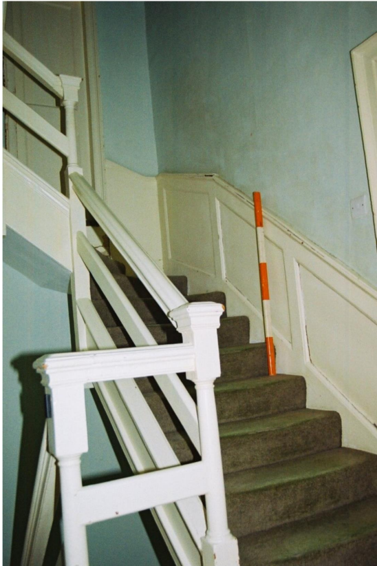
Figure 4 1730 Back Staircase at second-floor level with inserted guard rail (F1:30)
