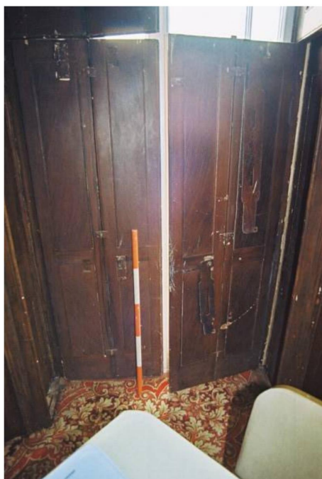
Figure 14 The shutters of the east range windows (east side of bay windows; F1:10)
