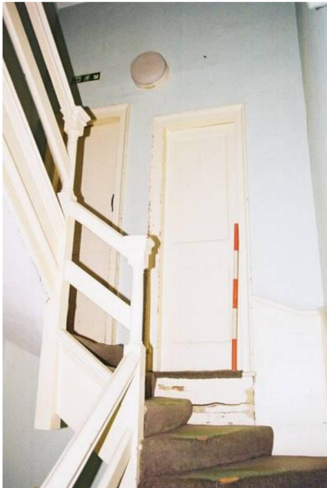
Figure 20 Doors for servants' ?closets below the eaves (F1:30)
