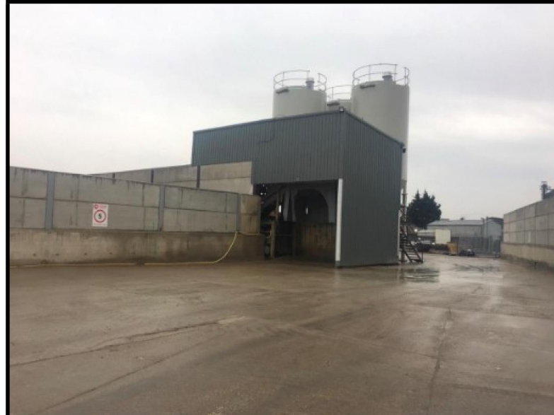
Figure 6 – View of Building and Concrete Storage Silos at Bexley Depot
