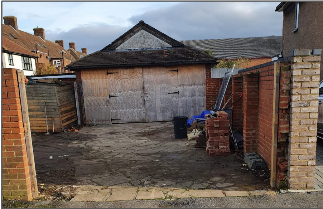
Figure 1: The Site -composed of concrete hardstanding and garage.
