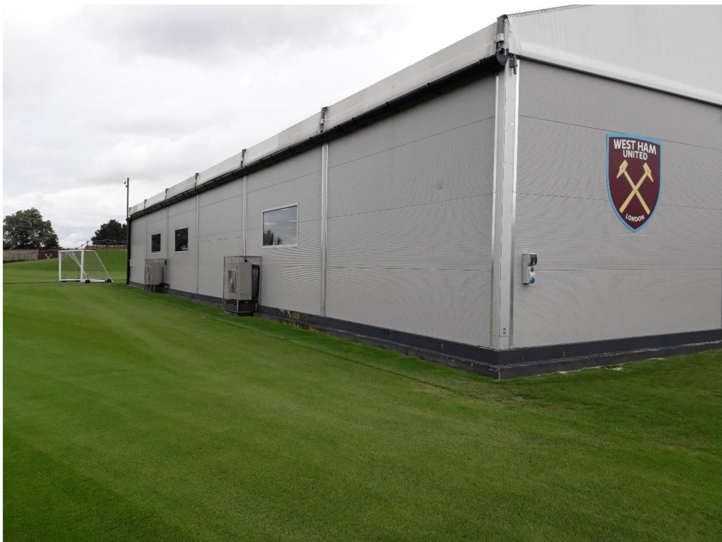
View of temporary gym building from training pitches
