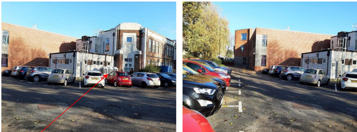
Figure 4: Drury Falls Building. Single storey part to be demolished under separate consent. Existing Ground level condenser units to be relocated onto the roof of BL1
