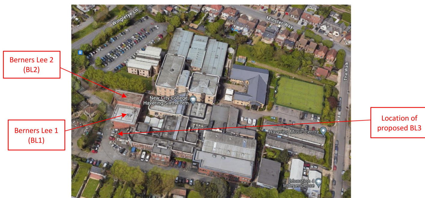
Figure 2: Aerial view of Wingletye Lane Campus and location of Berners Lee 1, 2 and 3
