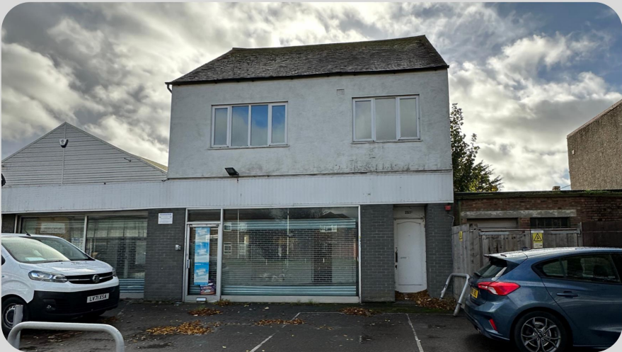
251 London Road, Romford, Essex RM7 9NJ - Front View
