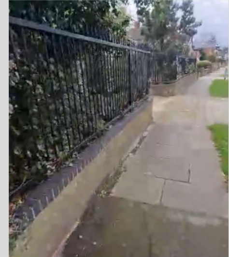
No. 22 Nelves Crescent
