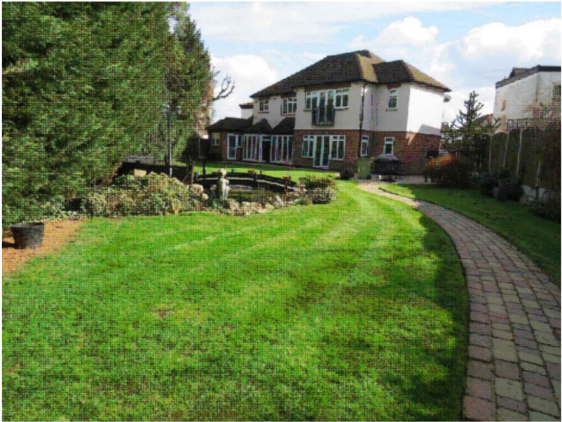
PHOTO-Existing rear elevation
