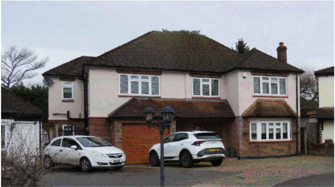
PHOTO-Existing front elevation
