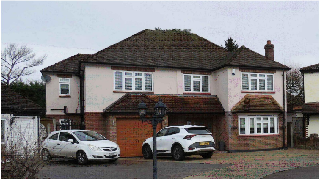
PHOTO-Existing front elevation
