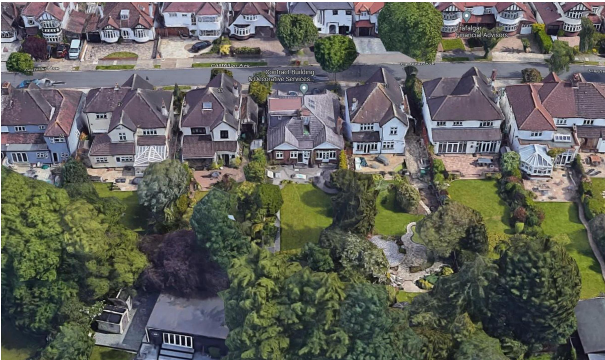
Figure 3 Shows the application site from high level rear.
