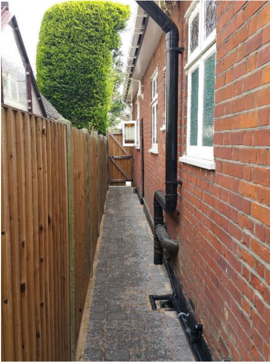
Figure 6 Showing photo of existing side wall face brickwork which the proposed flank walls will match.
