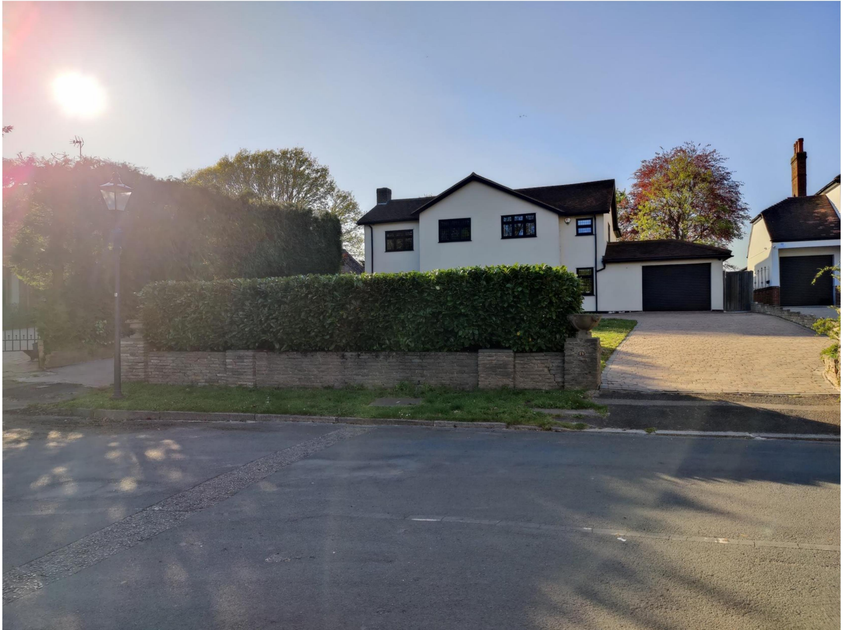
Image 1.0: View of the house from the road
