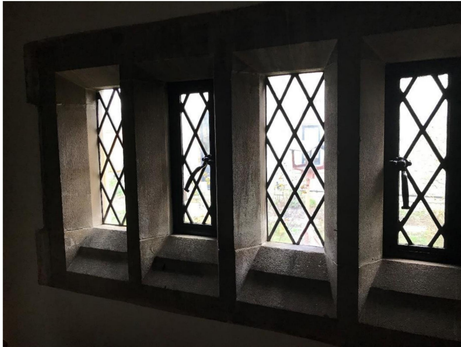
Figure 25: Detail of mullioned window to the Reconciliation Room / Confessional
