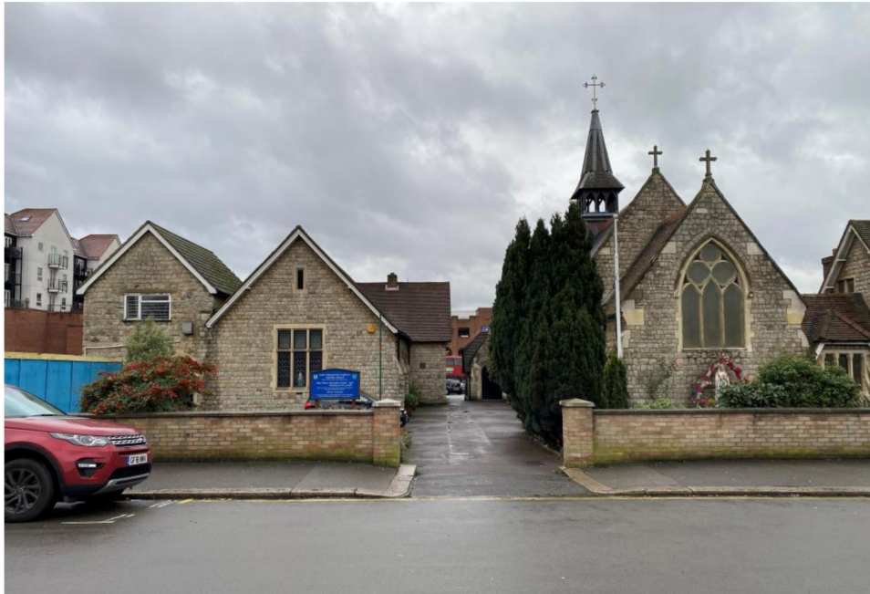
Figure 15: The application site looking west from Park End Road
