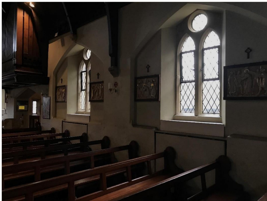
Figure 26: View north from the nave of the Church. The windows would potentially be partially blocked / occluded by an extension on the east side of the Lady Chapel
