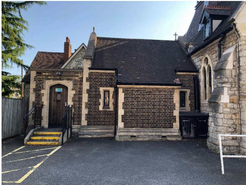
Figure 3: Lady Chapel viewed from the west side of the Church
