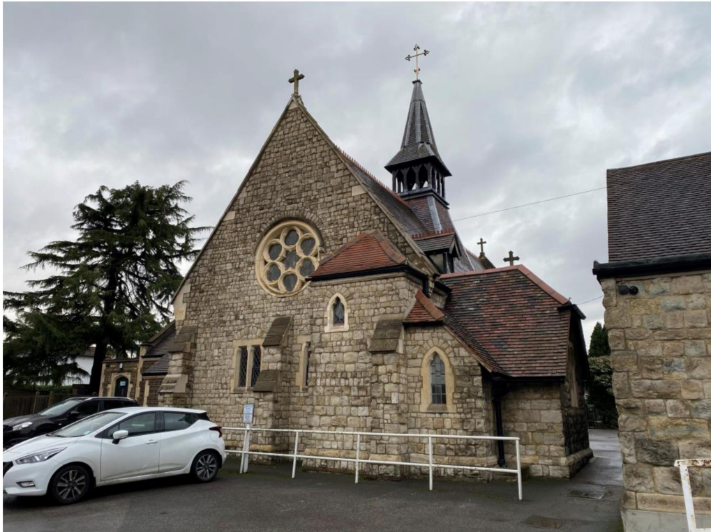
Figure 23: West elevation of the church
