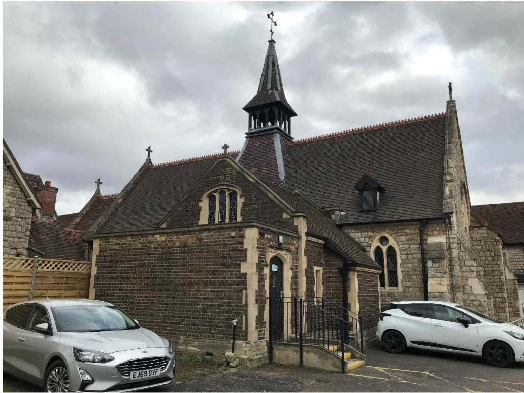
Figure 21: Close range view of St Edward's Church and Lady Chapel (to left)
