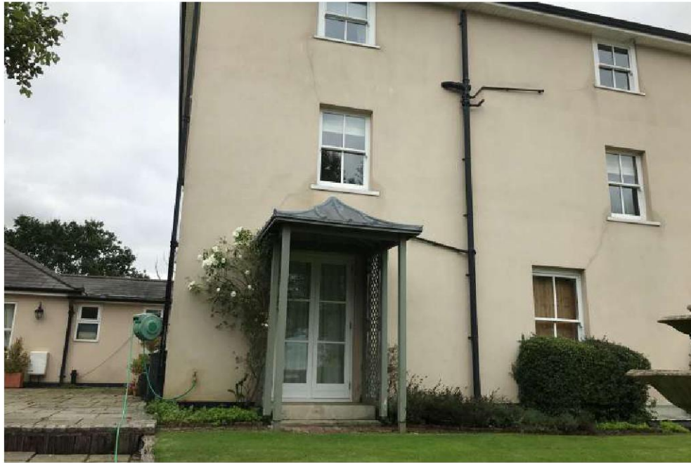
Further photo of Moor Hall.
