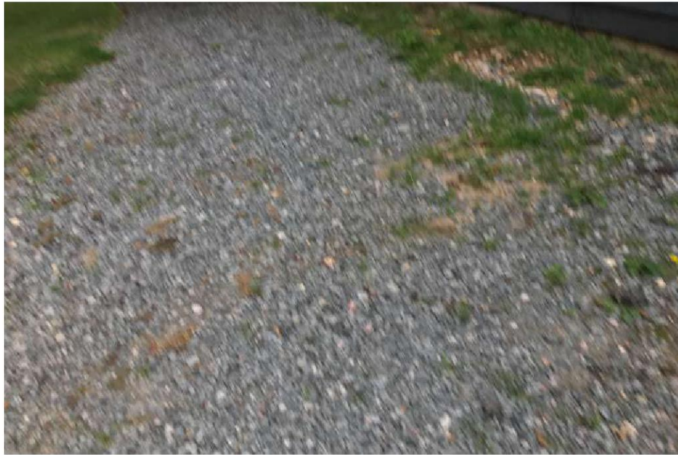
Photo of gravel surfacing in south of site.
