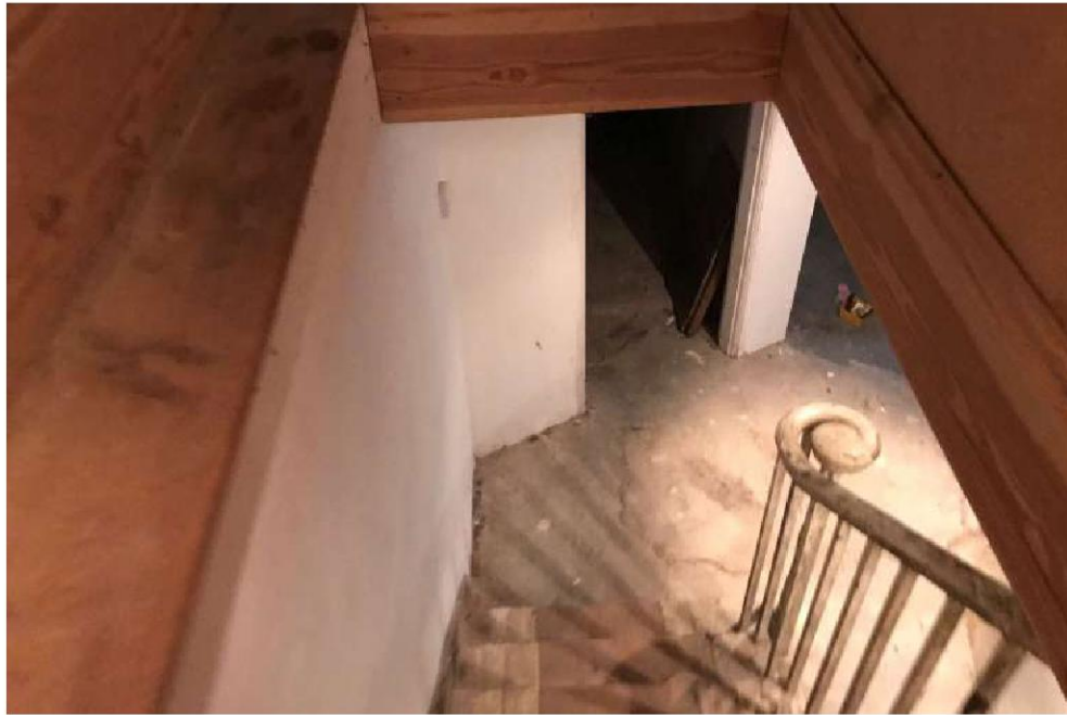
Basement of Moor Hall.
