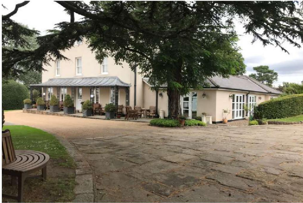
Photo of Moor Hall looking south-west.
