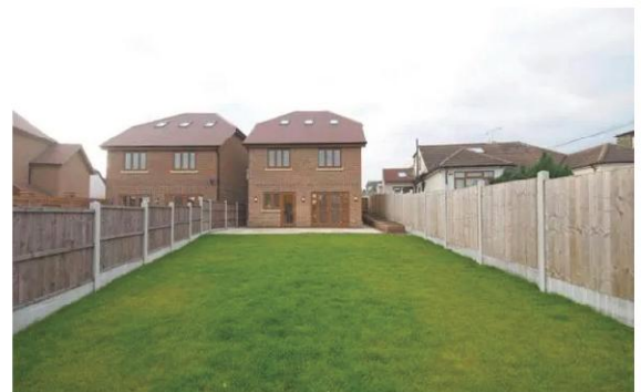
^ VIEW OF PROPERTY FROM REAR GARDEN
