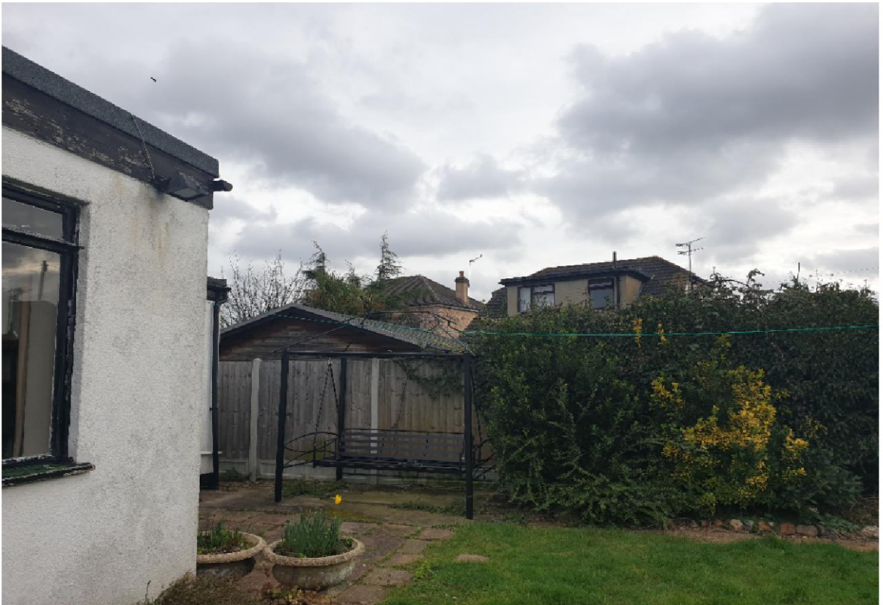
5 - REAR LOOKING TOWARDS 113 & 111 MOOR LANE
