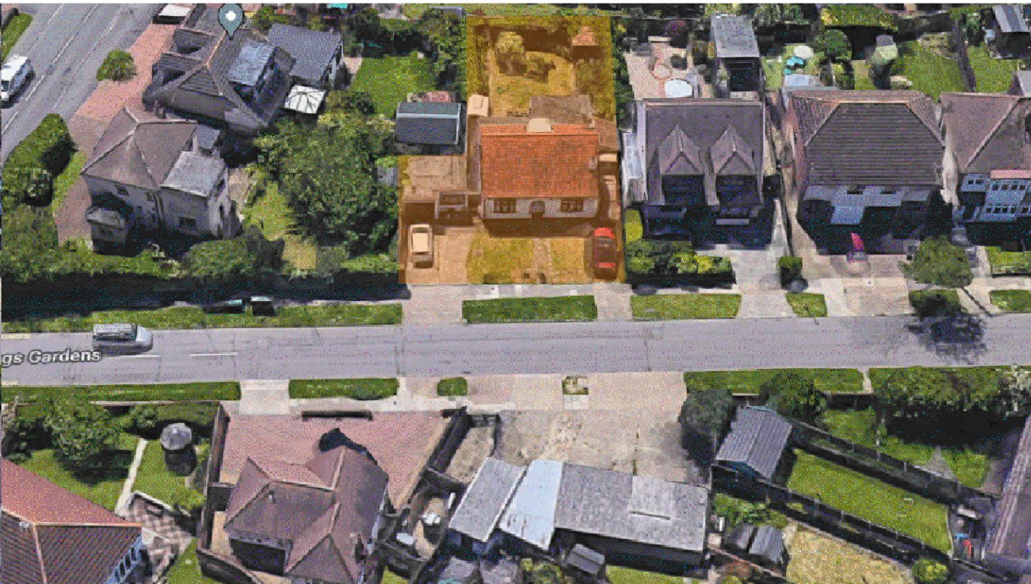
ELEVATED FRONT VIEW
