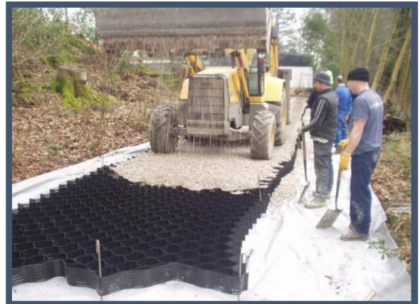
Figure 11 Examples of Cellweb filling with angular stone
