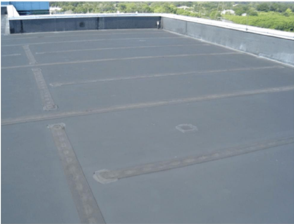
Flat Roof Type 1: Single Ply Membrane Roof
