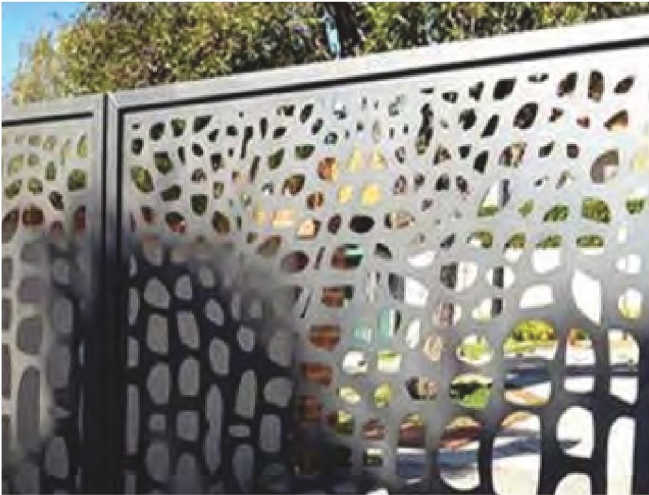
Main Entrance Gates: PPC pattern full height gate. PPC laser cut pattern.
