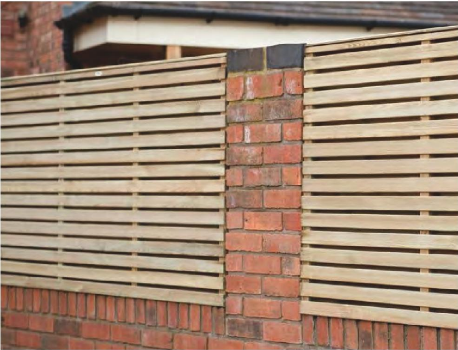
Boundary Fence Type 2: Brick wall + timber featherboard
