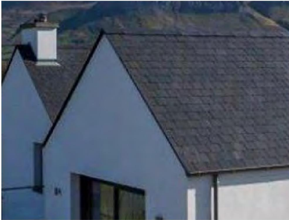
Pitched Roof: Fibre cement slate
