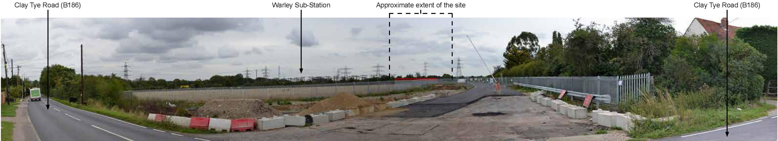
PRINCIPAL VIEWPOINT 3: VIEW FROM CLAY TYE ROAD (B186) LOOKING EAST TOWARDS WARLEY SUB-STATION
