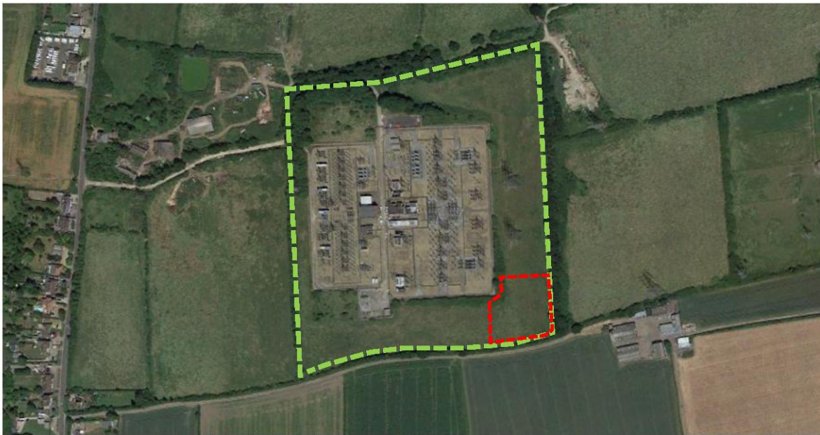
Figure 3 Aerial photograph of site with boundary. Substation curtilage highlighted.
