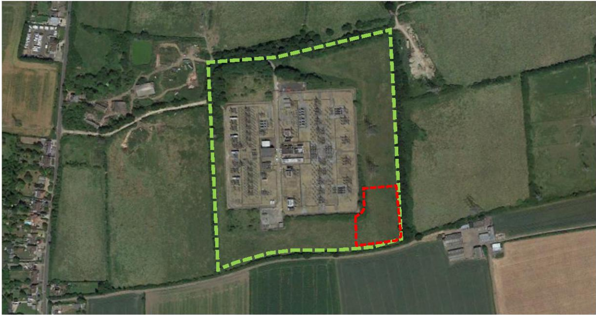
Figure 3 – Warley Electricity Substation with curtilage highlighted green
