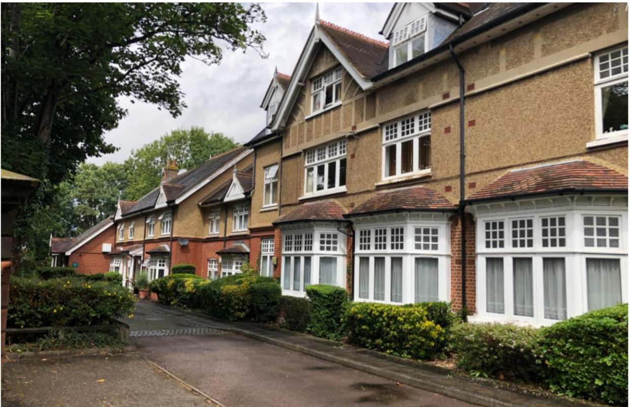
Figure 2: Existing South West Elevations / Side (June, 2020)
