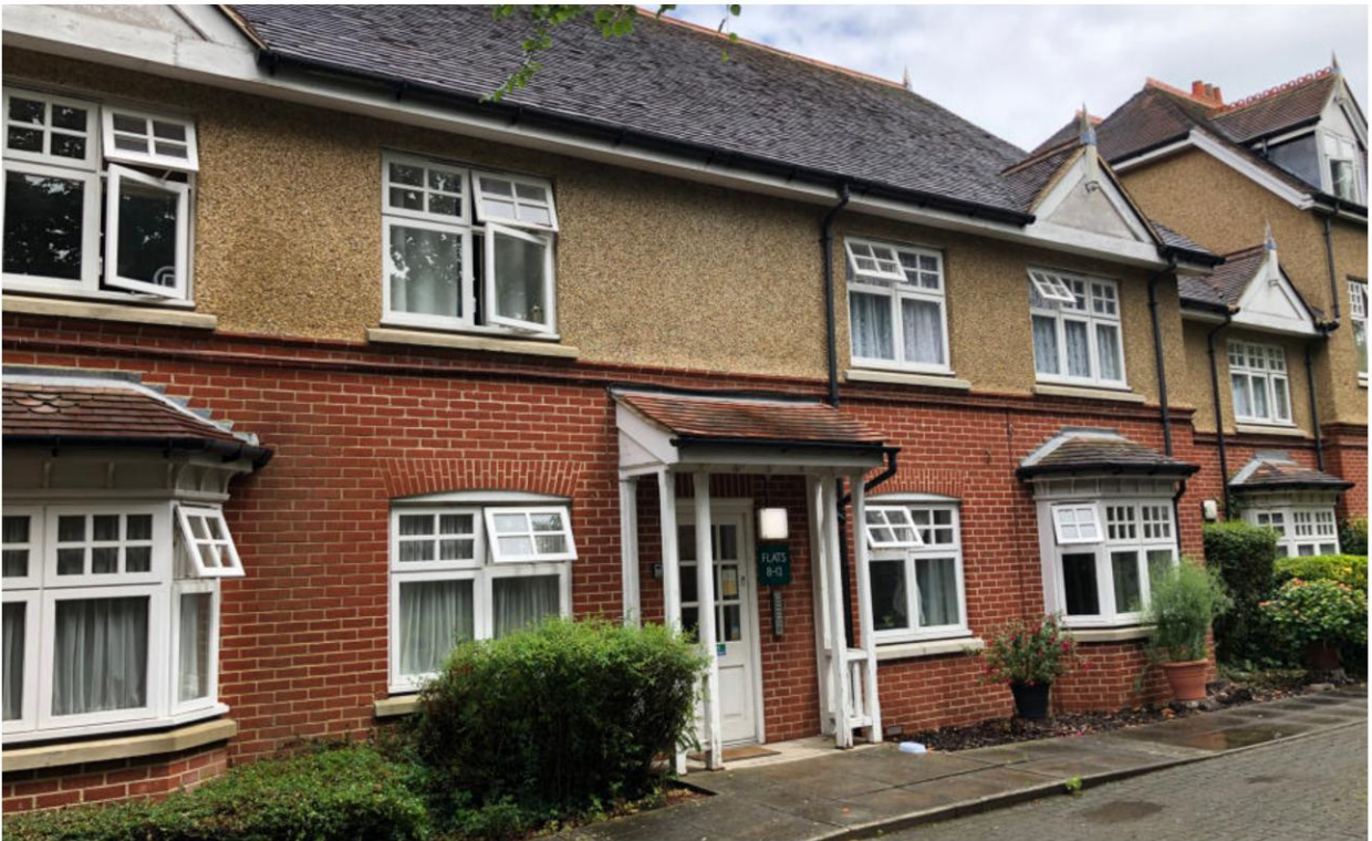
Figure 3: Existing South West Elevations / Side (June, 2020)
