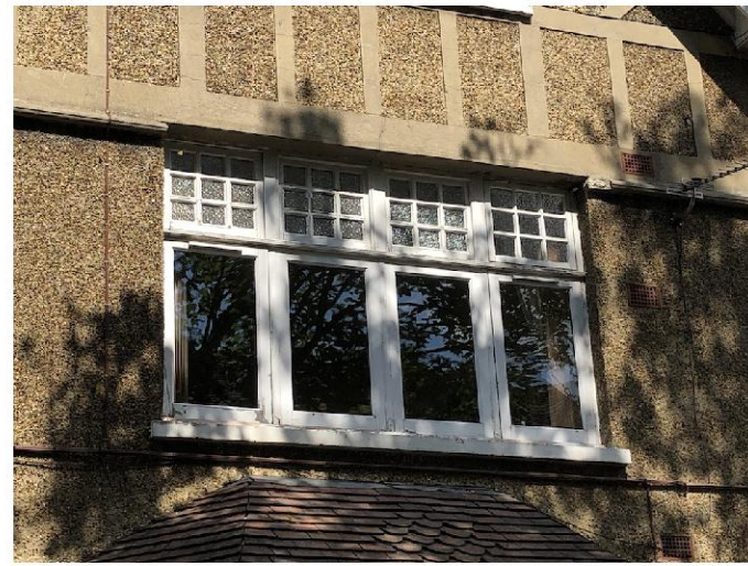
(B) Existing Bay Elevation and extract of existing timber casement window
