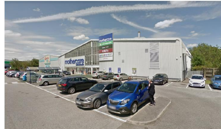
Figure 3: View from Car Park to Existing Front Elevation
