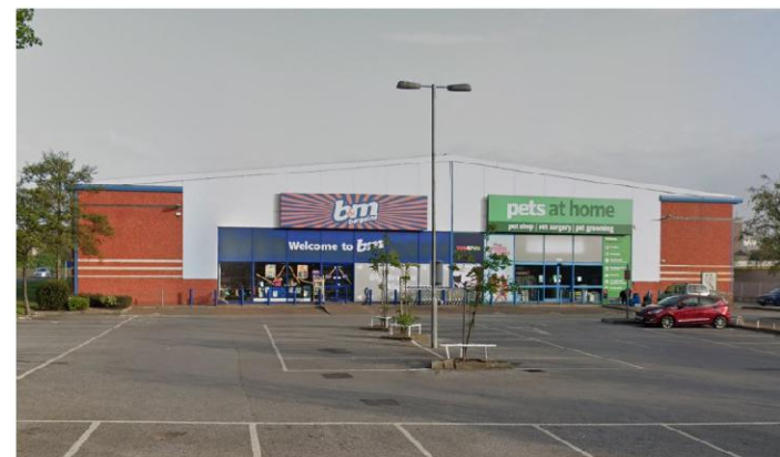
Figure 4: View of B&M and Pets at Home Stores Across the Access Road
