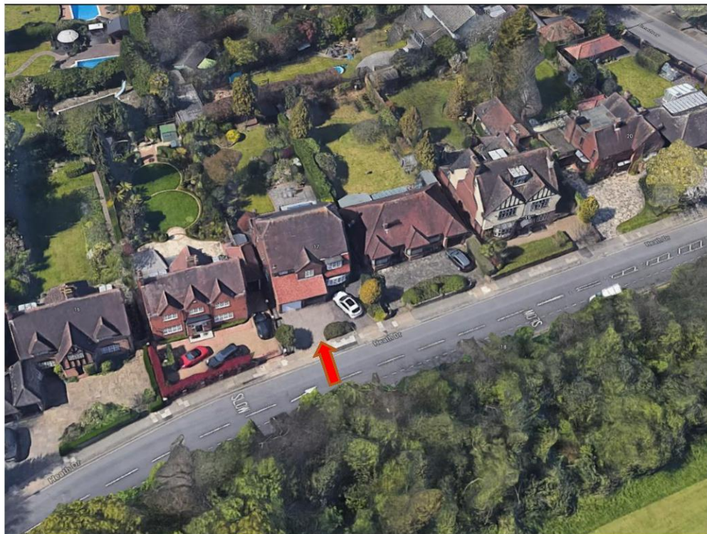
Aerial view of the application site (shown with red arrow)
