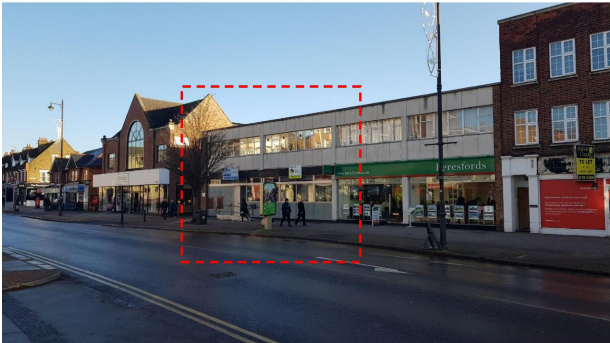
Station Road Streetscape
