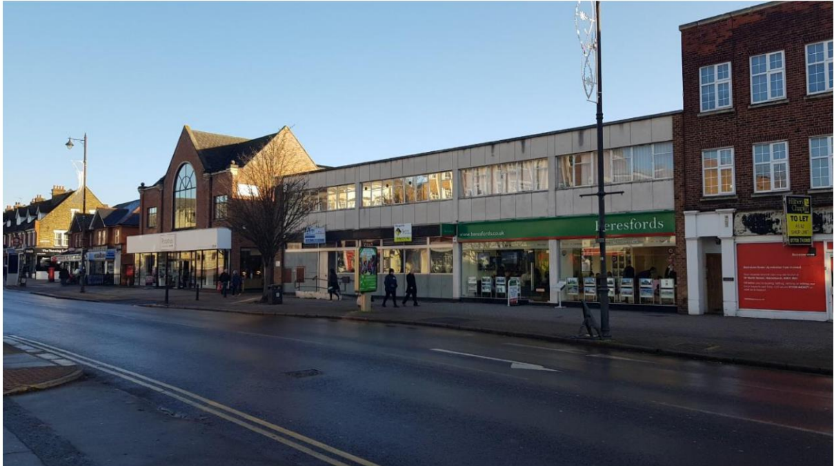
Photo of existing front elevation and relationship to adjacent buildings.
