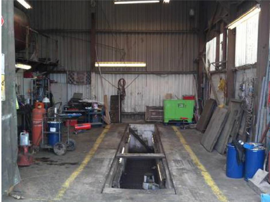
Looking southwest inside the existing workshop, which will be the location of the new tipping shed.
