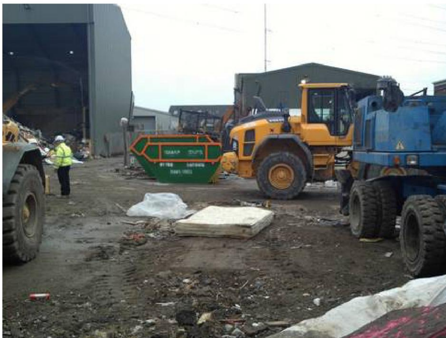
Looking southwest across the north area of the site used as yard storage, which will be the location of the new maintenance building. The existing workshop building is in the background and the adjacent existing main recycling building is in the background on the left.
