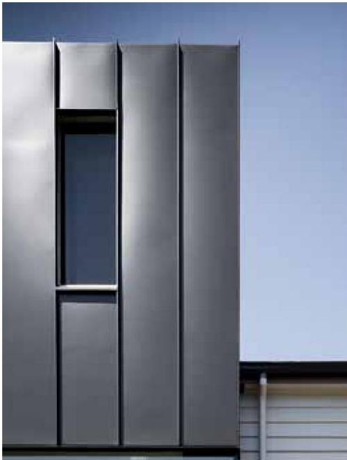
Vertical standing seam metal cladding
