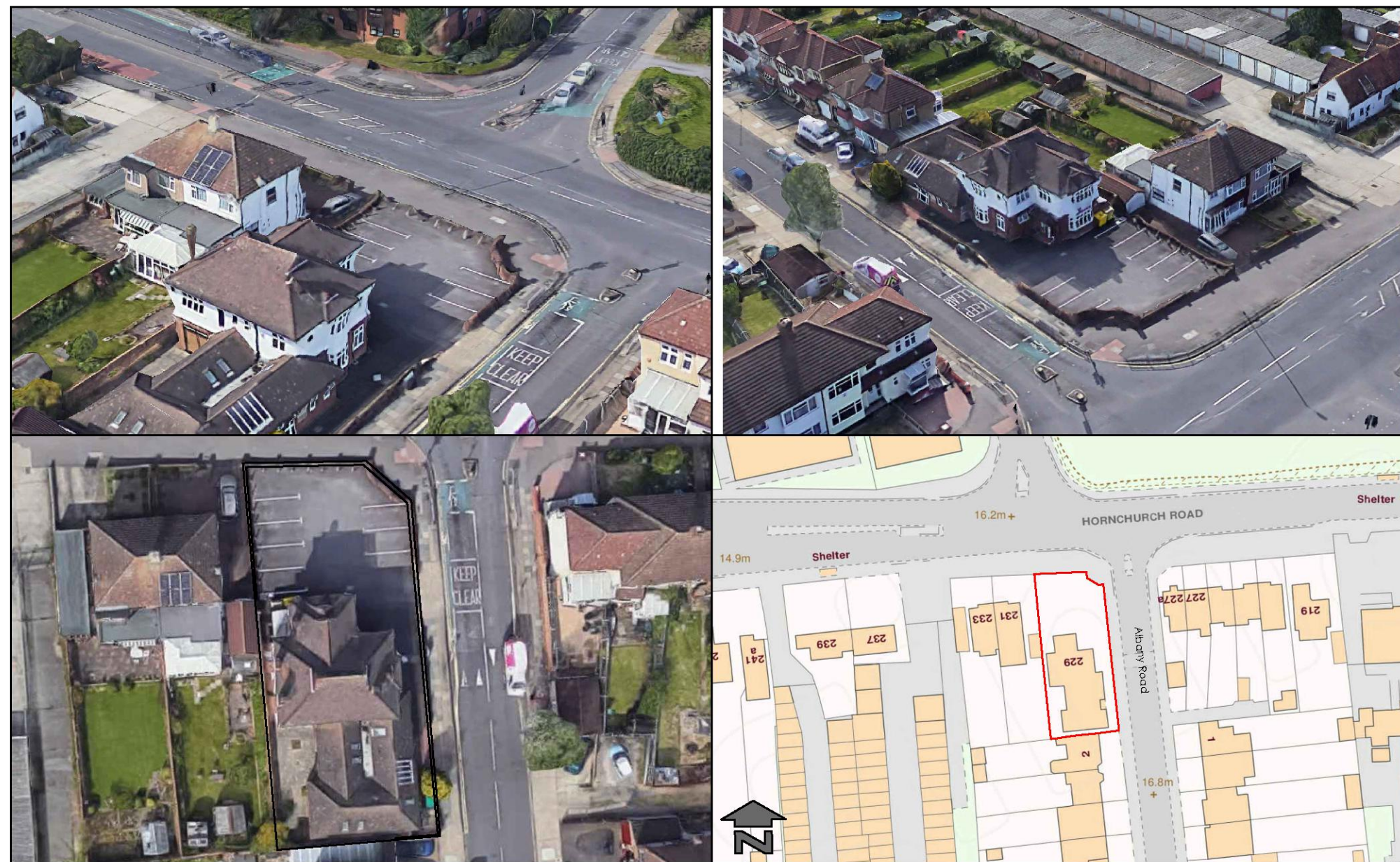
08 AERIAL PHOTOGRAPH SCALE N/A
